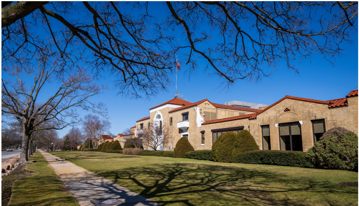
Top: Mars Candy Factory after completion, 1929. Source: Mars, Inc. Bottom: Mars Candy Factory, 2023.
