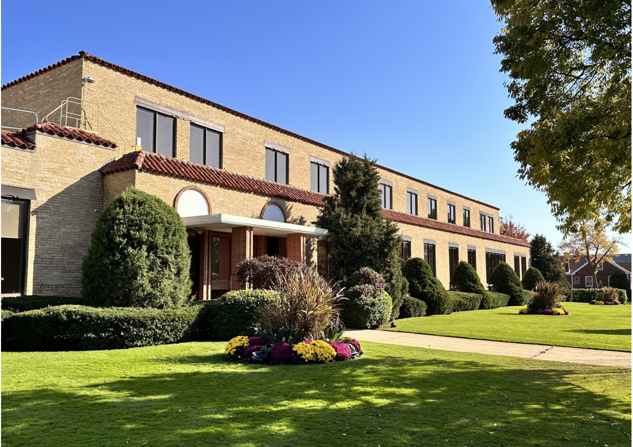
The 1960 two-story office addition designed by C.F. Murphy Associates.
