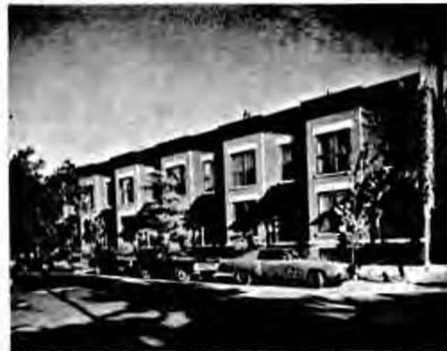
These row houses are typical of the kind that began to appear in the late nineteenth century, giving Mid-North an urban character.
