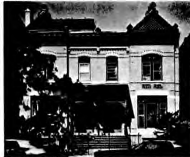
These town houses display the rich variety of color and texture found on Queen Anne facades. Note the use of leaded glass in the windows.
