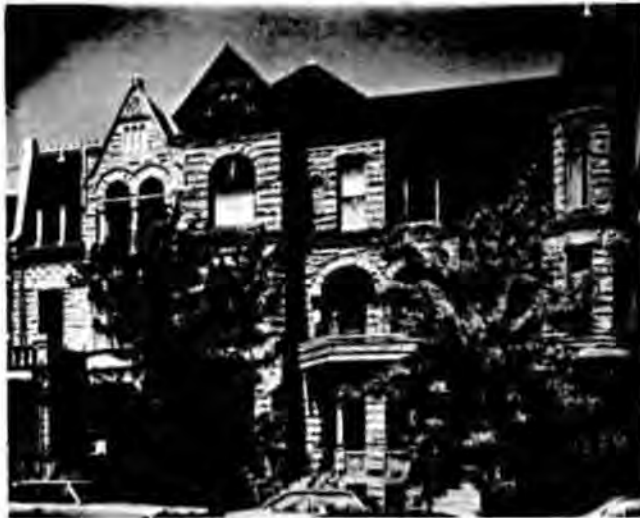
The building at 540 Belden Avenue ( right ) displays the arched window openings and rough faced masonry facade characteristic of the Richardsonian Romanesque.
