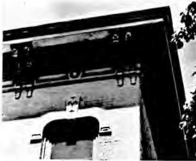
This boldly projecting cornice with elaborately carved brackets is typical of the Italianate Style.
