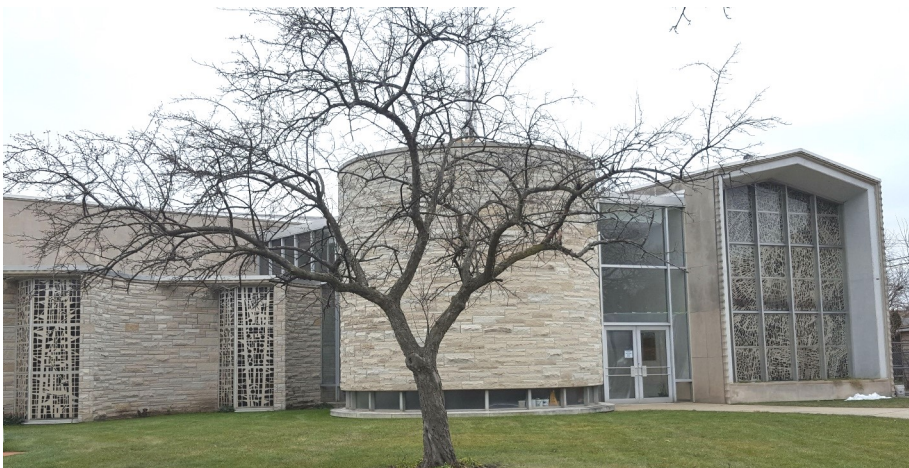
The raffle succeeded in raising funds for the nearby St. William parish to build this church, as well as a new convent and rectory, also designed by Belli & Belli in 1957.
