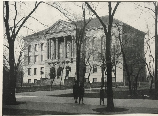
PATTON & FISHER, ARCHITECTS, CHICAGO, ILL.
