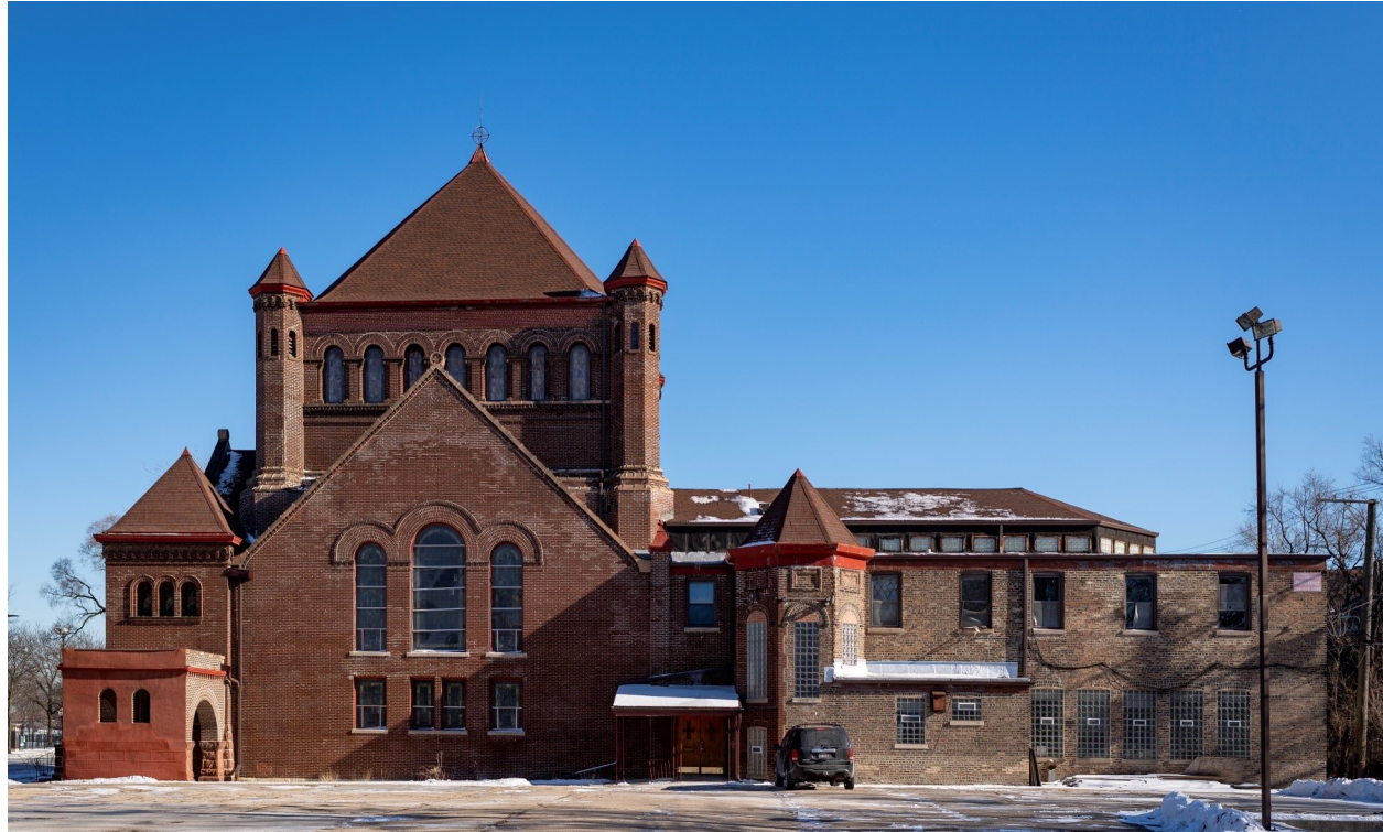
Then west elevation showing the Sunday School wing projecting to the rear of the church with its unusual clerestory. (Credit: Patrick Pyszka)
