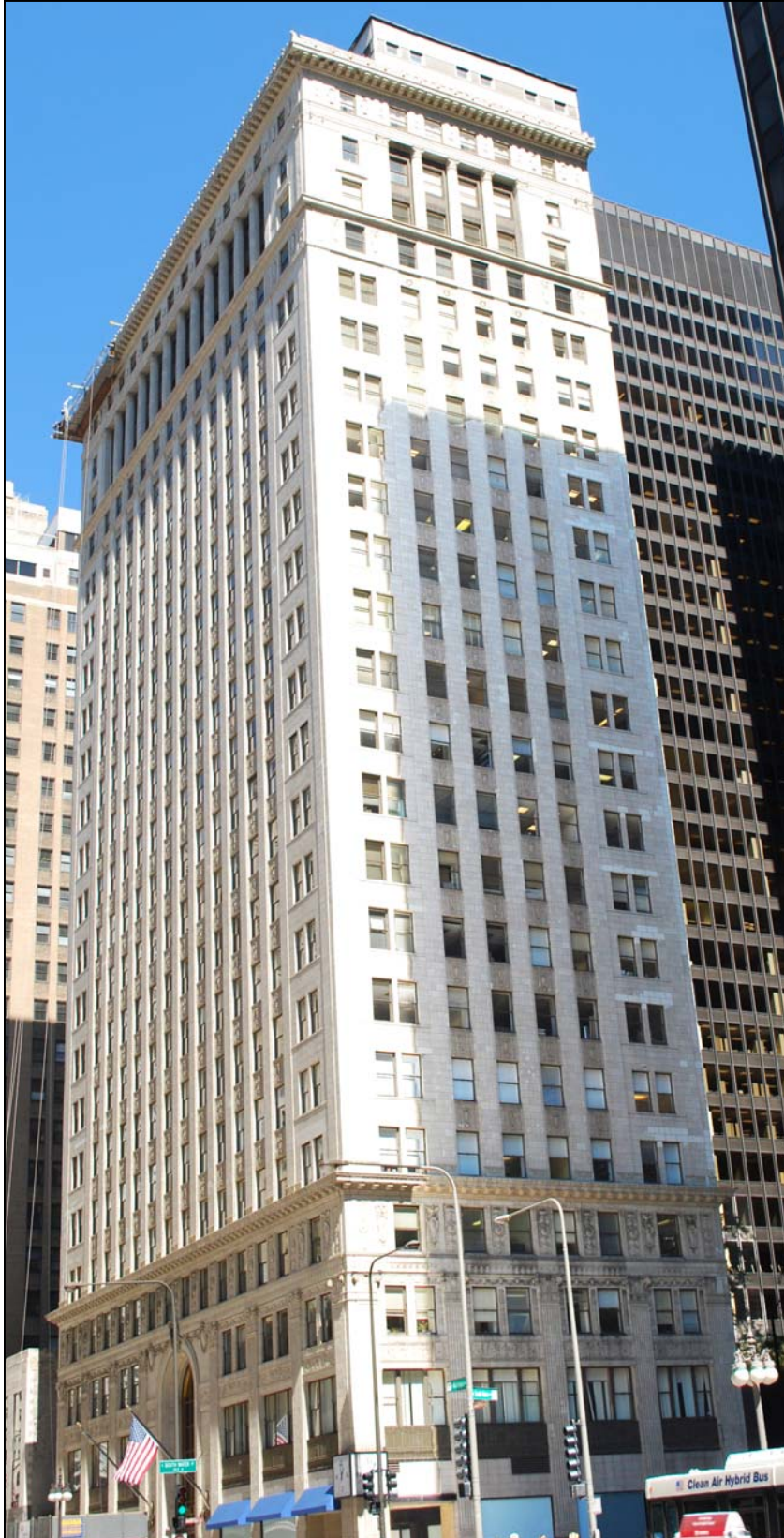
Left: The Old Republic Building viewed from the southwest in September 2010.
