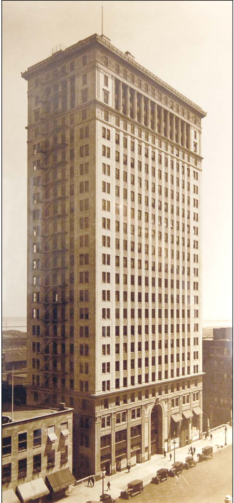
The Old Republic Building, ca. 1924, view from northwest.
