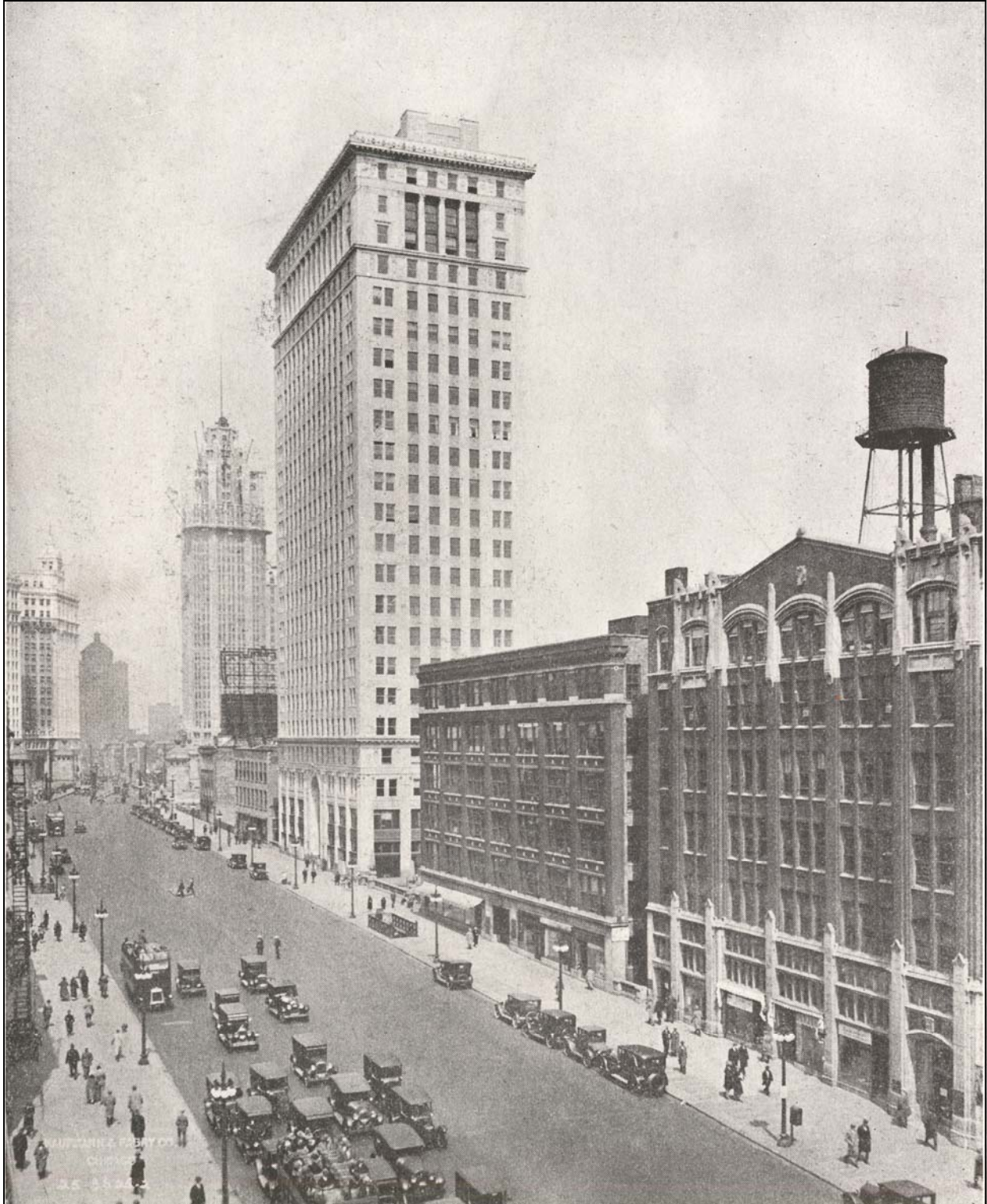
When constructed in 1924, the Old Republic Building was the tallest building on the east side of Michigan Avenue south of the river, and was visible for a great distance. At 264 feet tall, it was built to the full height allowed at that time by the Chicago Zoning Ordinance for a building without a set-back tower. Visibility was further enhanced by the bend in Michigan Avenue at the river, so that the Old Republic Building was centrally located on the avenue when viewed from the north.
