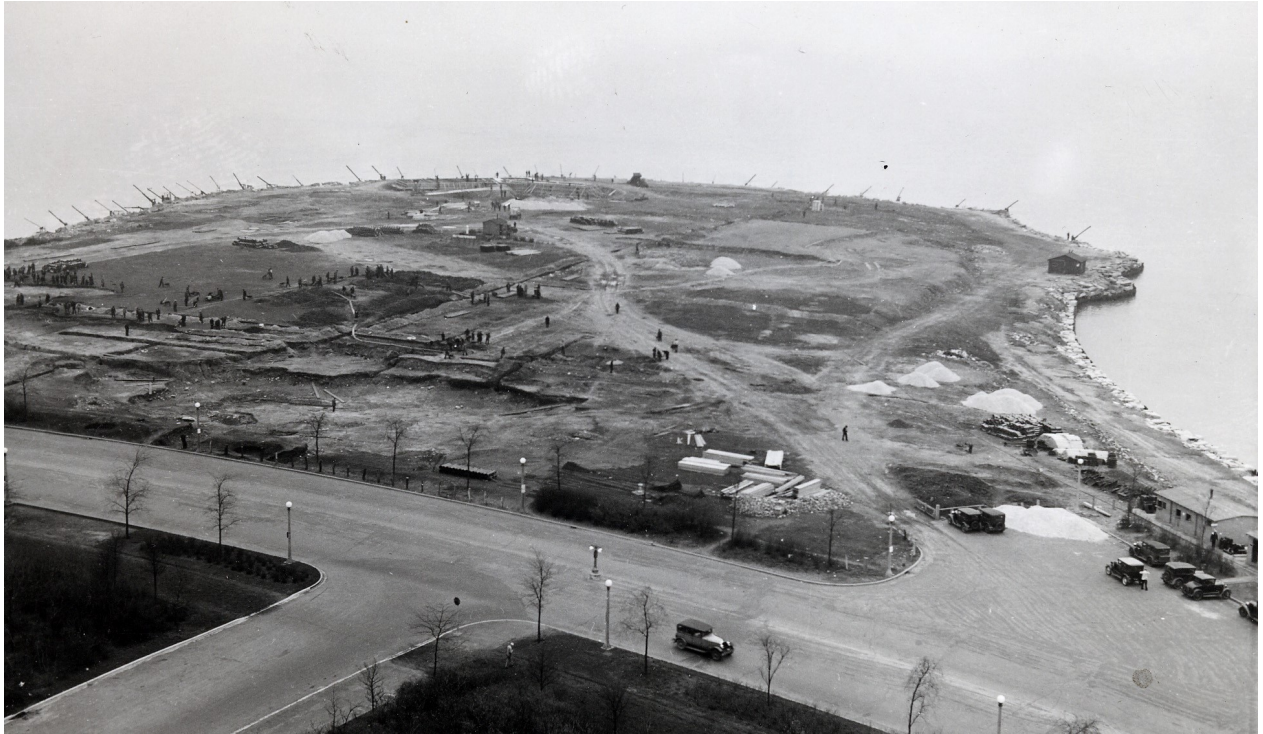
Above: Looking northeast toward Promontory Point, 1936. Work is underway to complete re- vetments and grading. (Source: Chicago Park District Records: Photographs, Chicago Public Library Special Collections)
