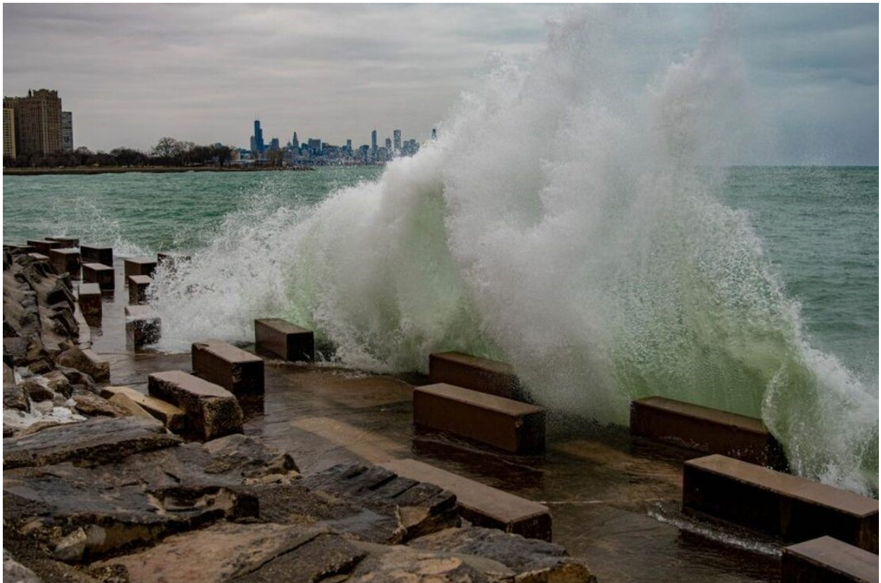
Below: In 1965, the stone platform from north of the pavilion around the east side of the peninsula was replaced with a concrete platform with almost ninety concrete deflectors. (Photo by Gabriel Issa; Source: U-High Midway online, April 6, 2022)
