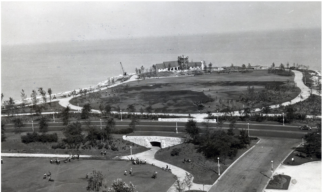
Below: Promontory Point, 1937. The underpass at 55th Street has been completed. The wings of the pavilion have been constructed and the tower is underway. (Source: Chicago Park District Records: Photographs, Chicago Public Library Special Collections)
