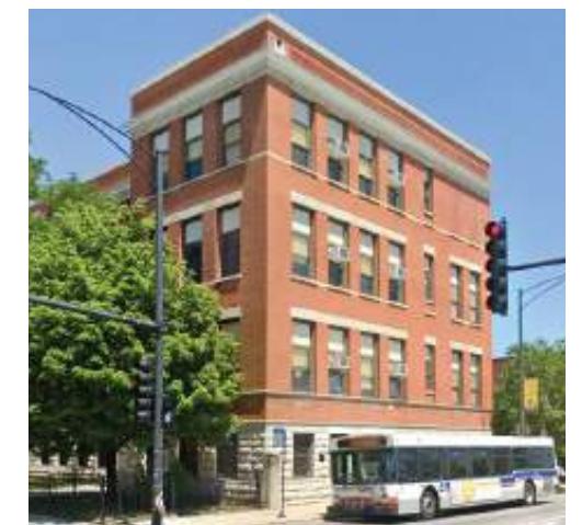
Figure 3-42: Curtis Elementary School at 115th Street and State Street Source: Google
