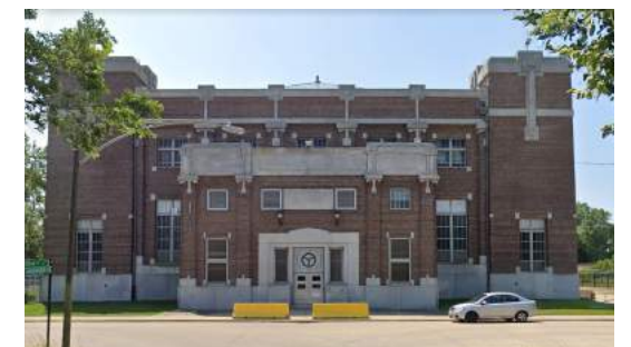
Figure 3-8: Roseland Pumping Station
