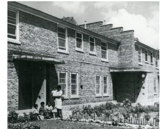
Figure 3-60: Historic Altgeld Gardens Rowhomes Source: Public Housing Administration / National Archives Catalog
