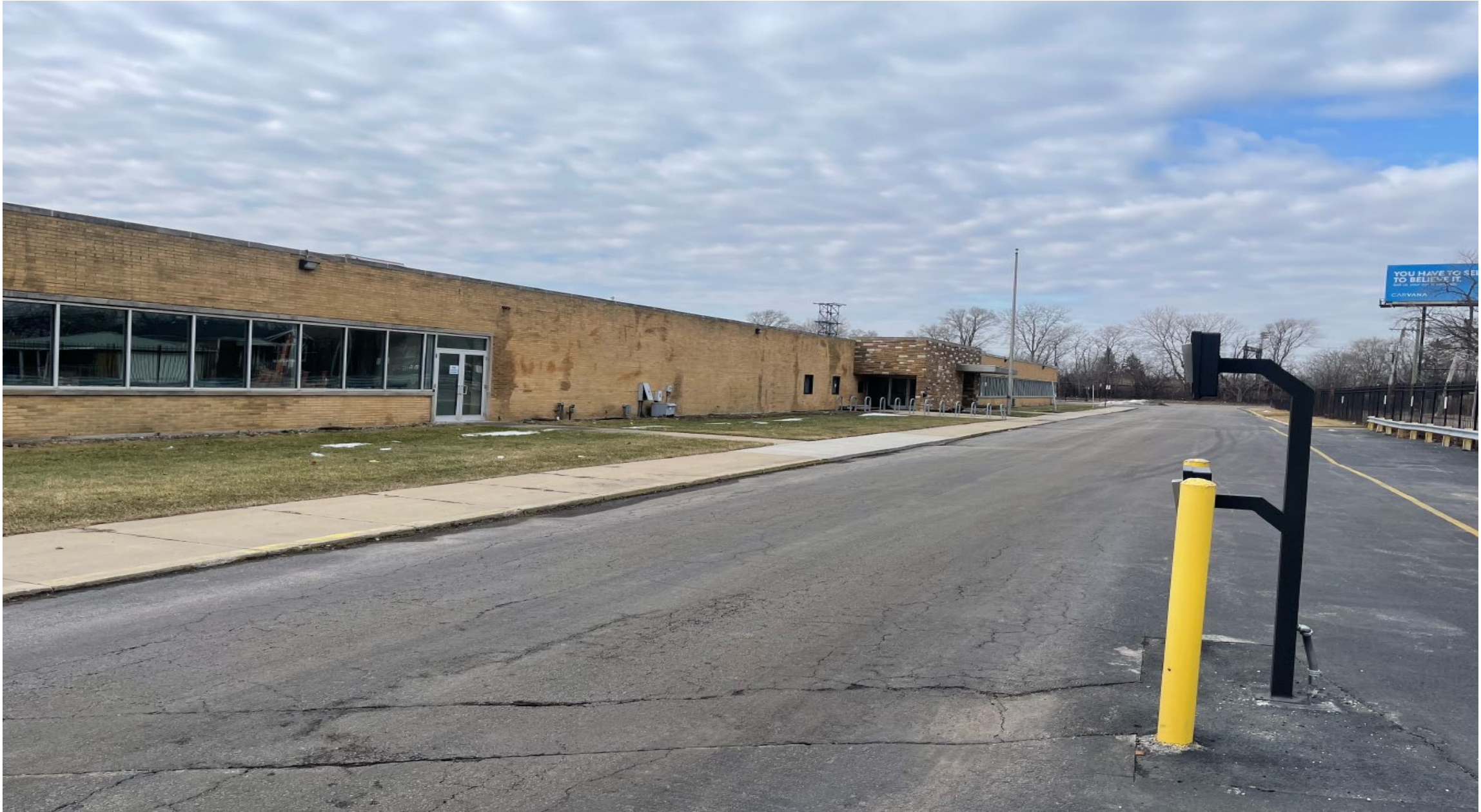
SITE CONTEXT: WEST VIEW OF SITE
