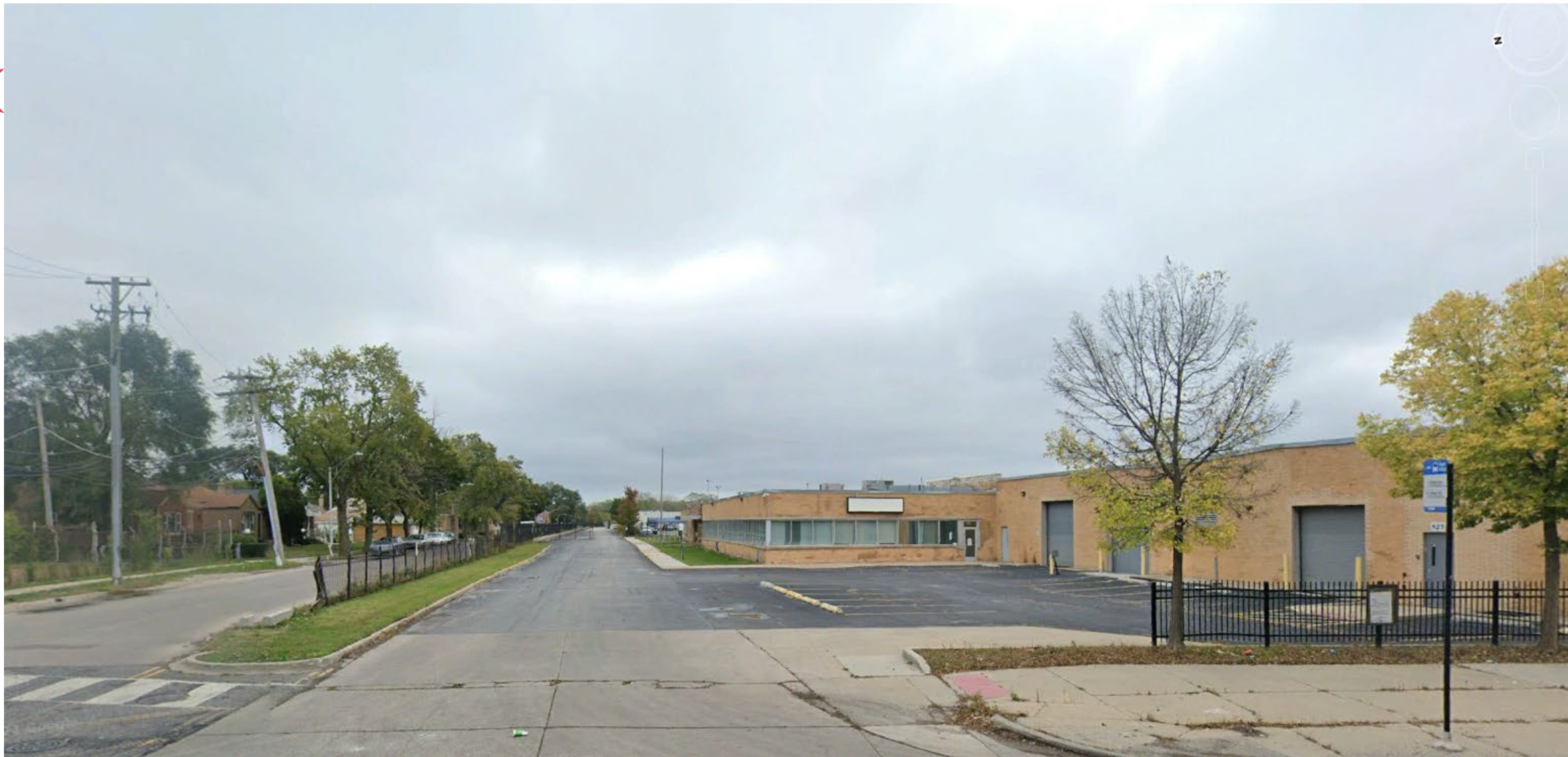
SITE CONTEXT: EAST VIEW OF SITE
