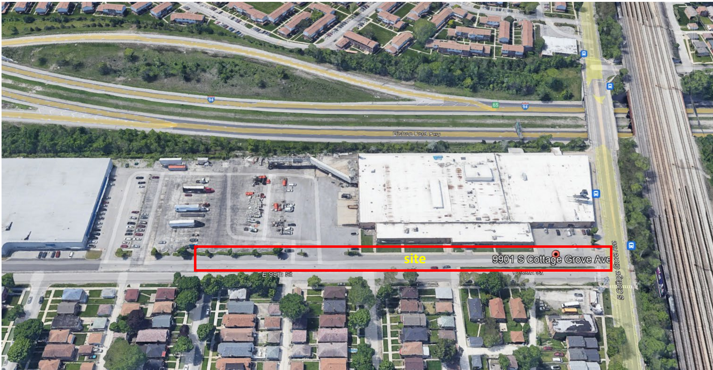
AERIAL VIEW FROM NORTH
