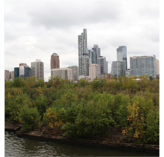
View of Site from Chicago River
