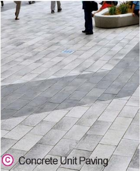
C Concrete Unit Paving
