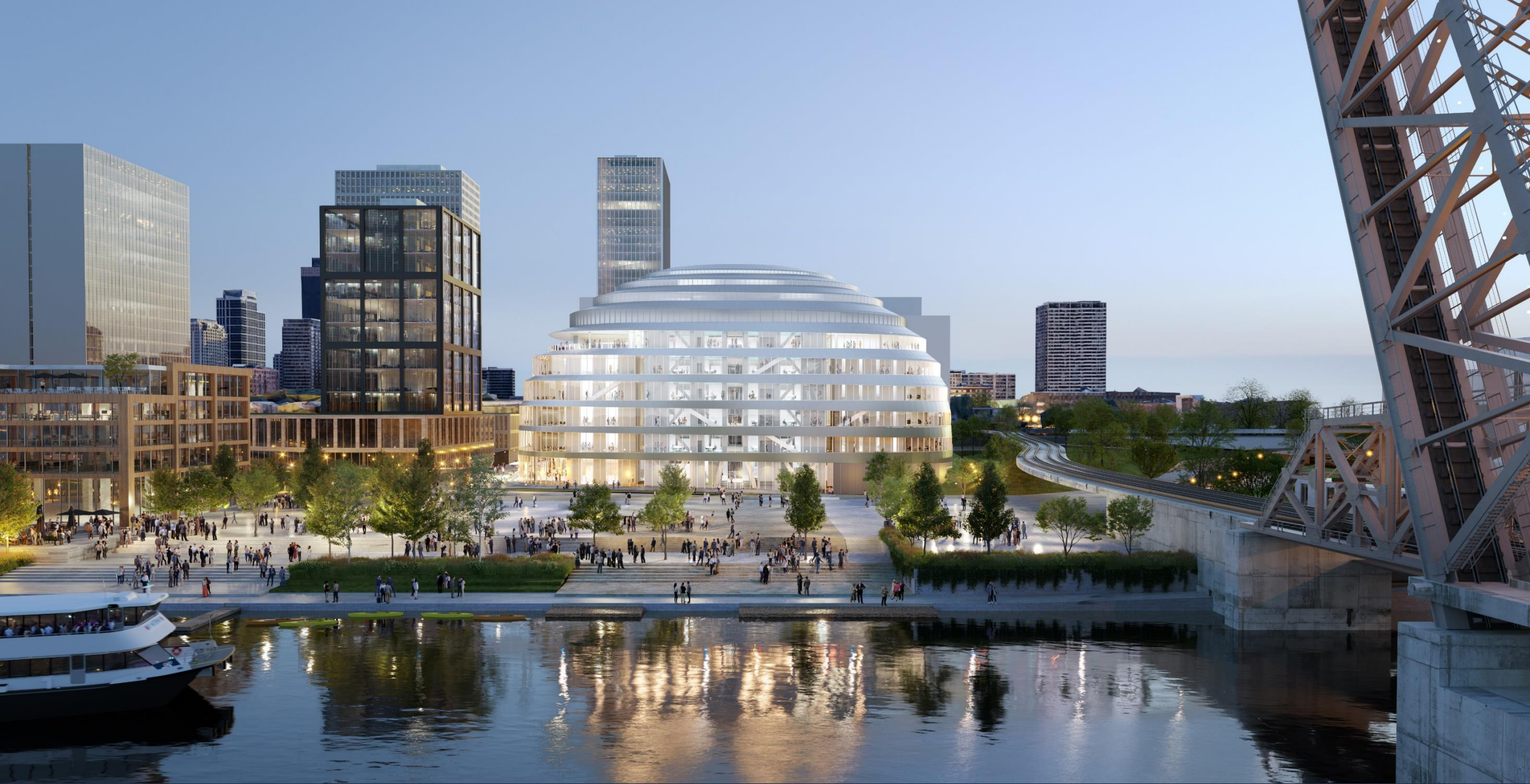
AERIAL VIEW FROM WEST DIRECTION
