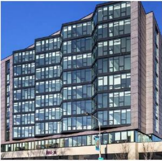
SAWTOOTH PROJECTED WINDOW BAYS
