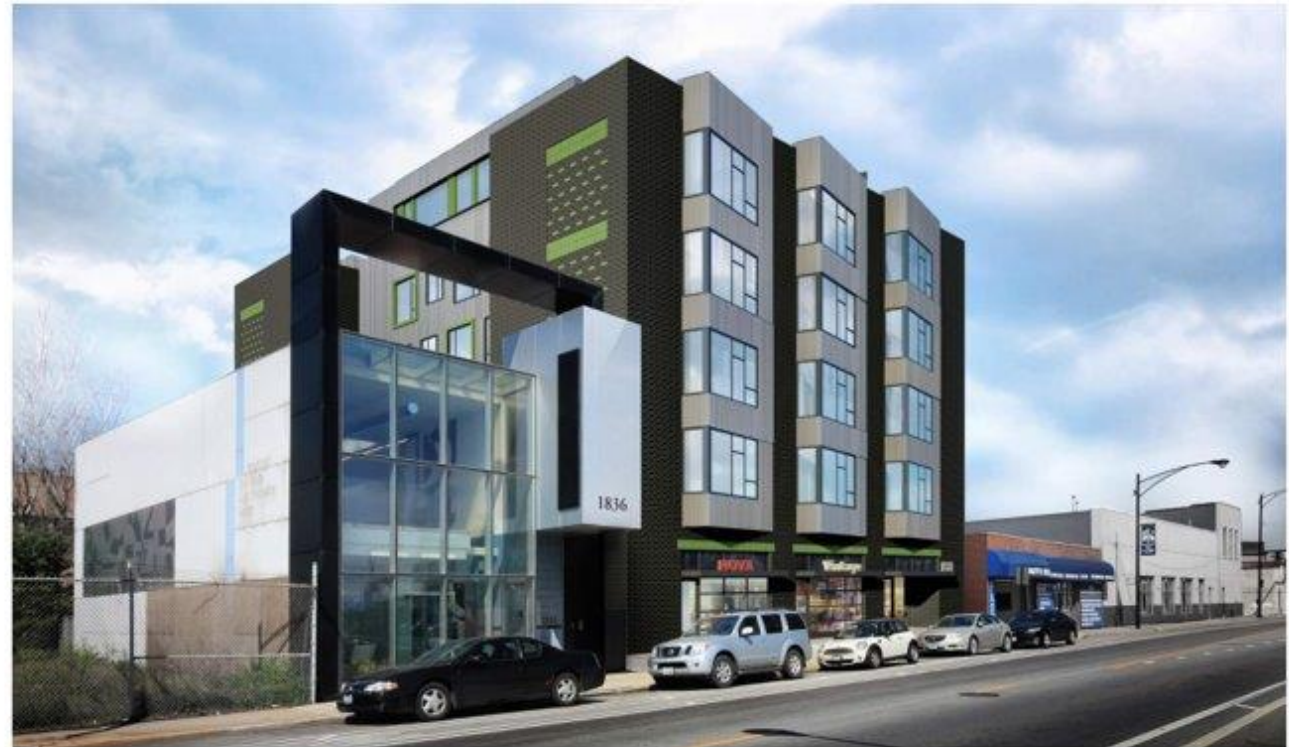
View Looking North along Elston Avenue
