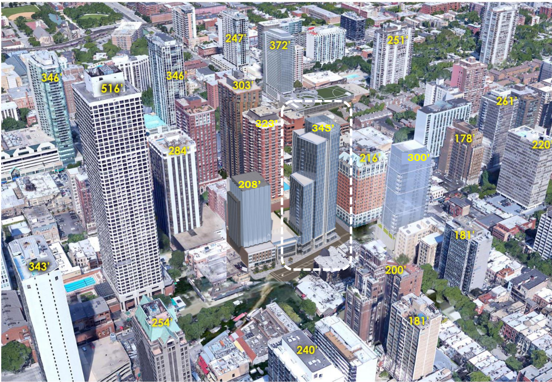
AERIAL VIEW LOOKING NORTHWEST
