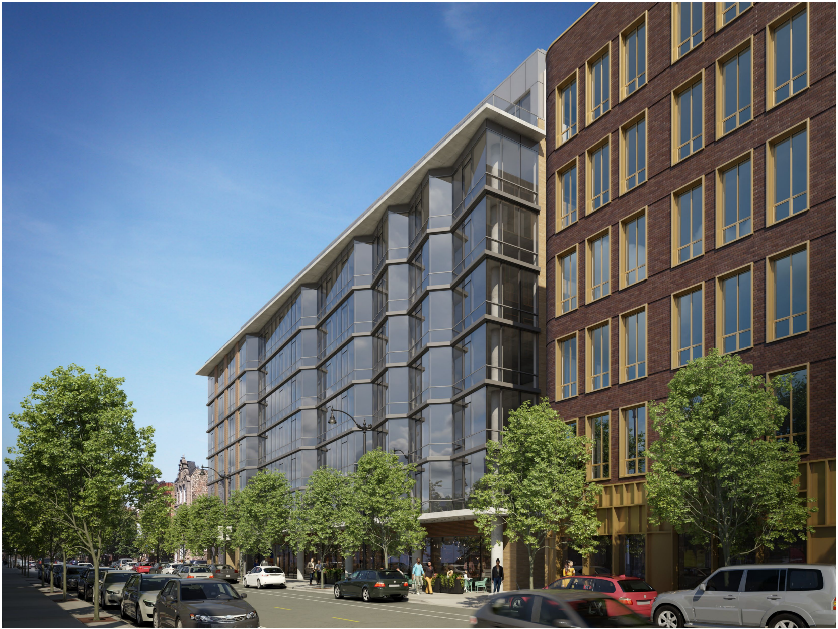
VIEW FROM SOUTHWEST ON HALSTED ST
