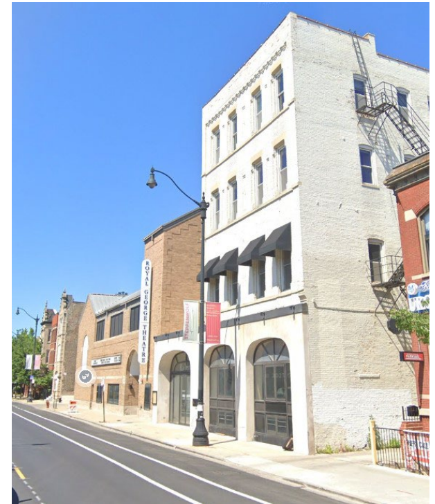
EXISTING VIEW FROM SOUTH
