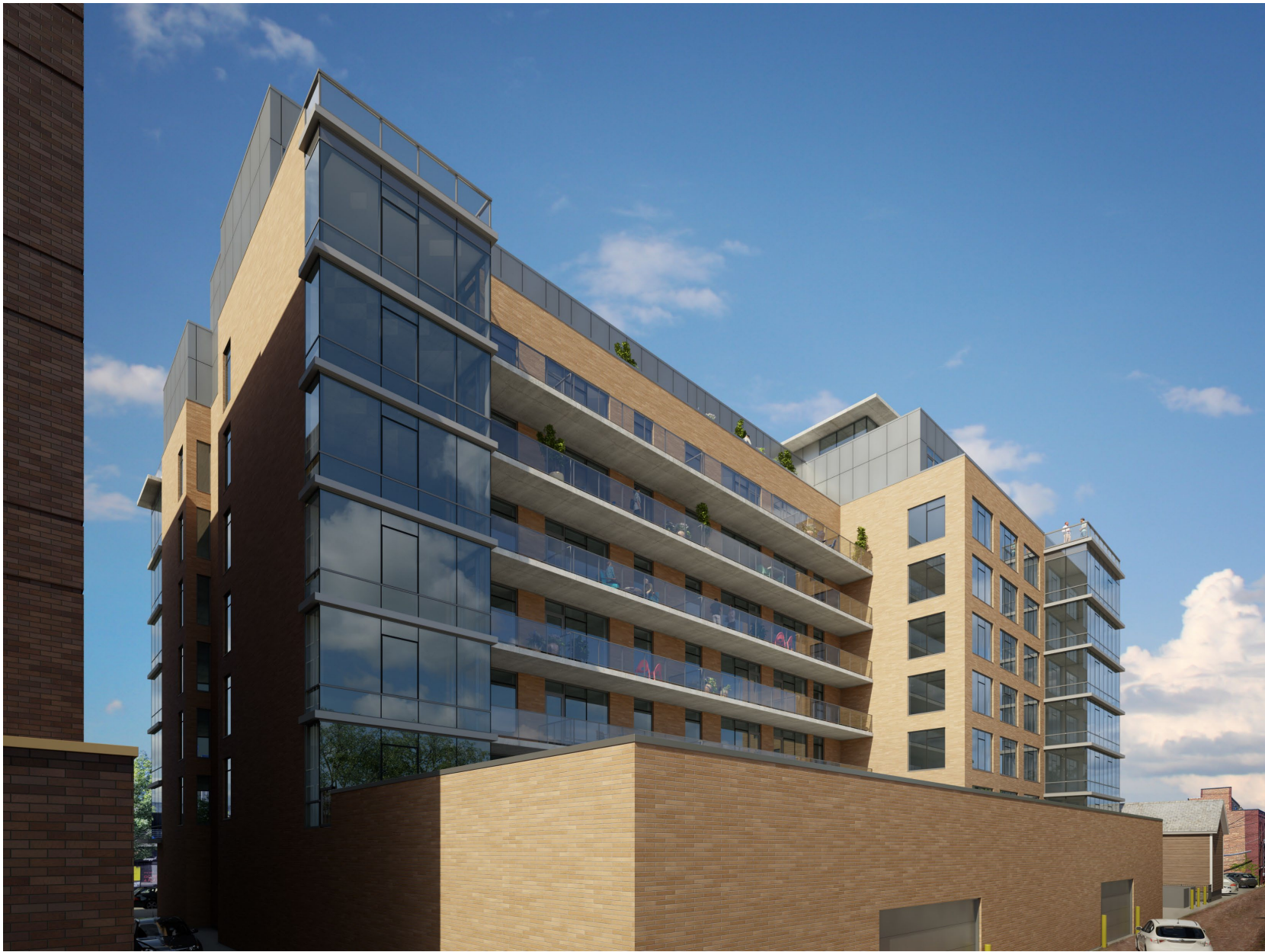
VIEW FROM SOUTHEAST IN ALLEY
