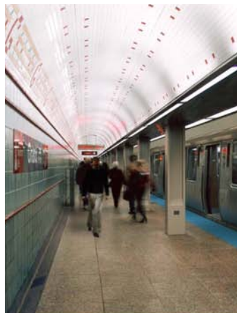
Image RN-6: Modernization of the Grand Red Line Station will improve platforms and mezzanines.
