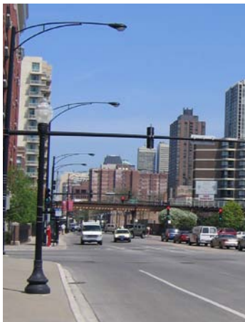
Image CA-6: The re-establishment of a CTA station at Division will improve access for Cabrini Area residents.
