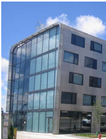
Image CA-3: The new Schiff Residences (Mercy Housing) along Clybourn through the Cabrini Area.
