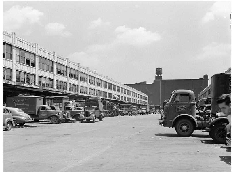
New South Water Market
