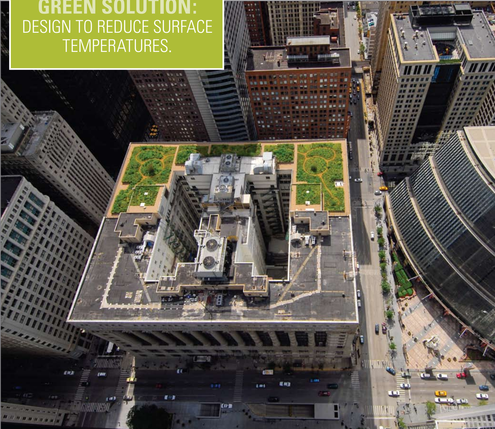
This recent photo of City Hall's green roof clearly shows the contrast between a vegetated and non-vegetated roof. The temperature differences between a vegetated and non-vegetated roof can be as much as 70 degrees.
