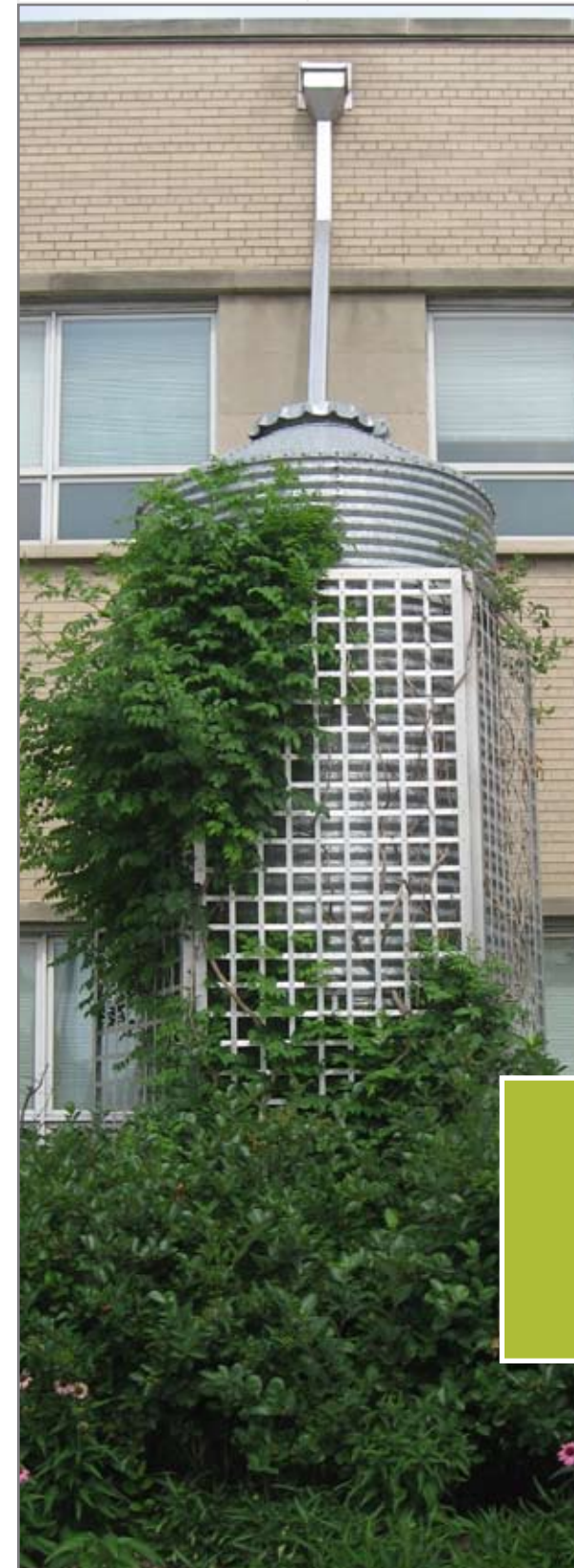
This 12,000 gallon cistern at the Chicago Center for Green Technology (CCGT) is covered in blooming vines, collects stormwater from the roof and stores the water for landscape irrigation.
