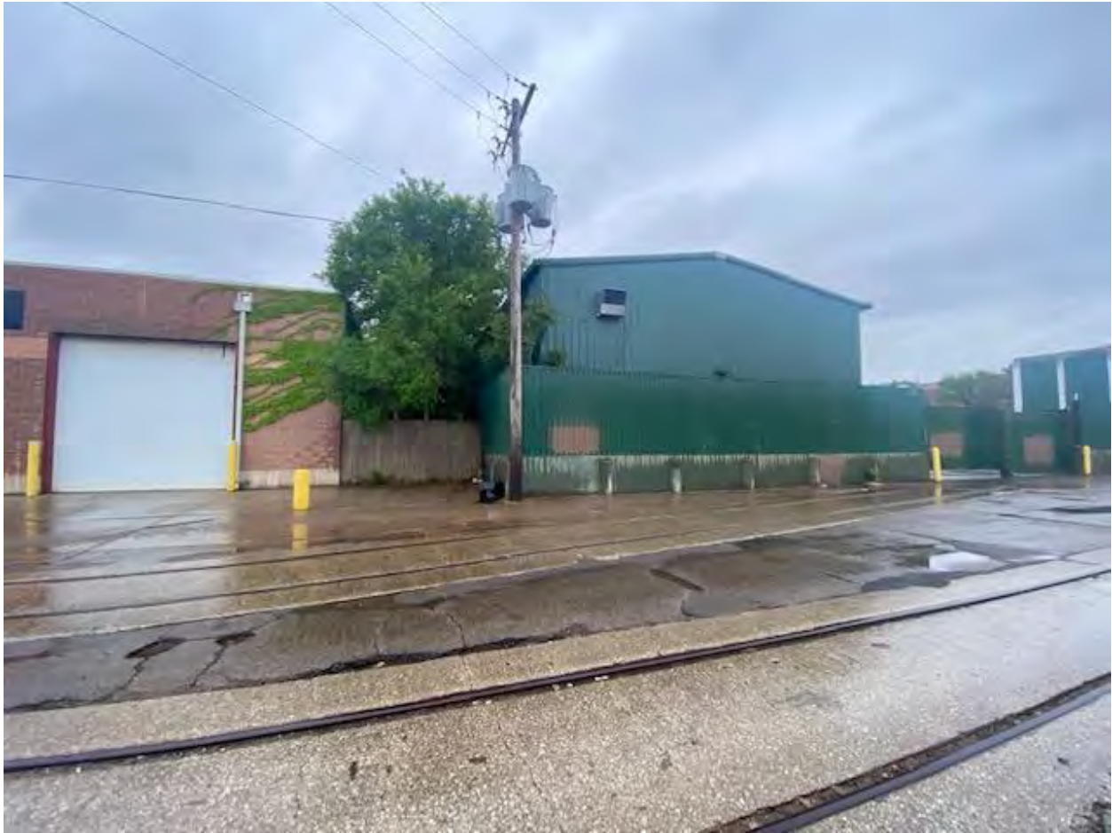
Photo 1 Existing pre-engineered metal building wall along east elevation
