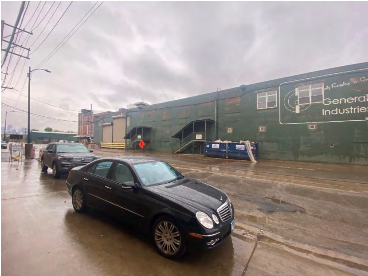
Photo 1 Existing Brick bearing wall along south face
