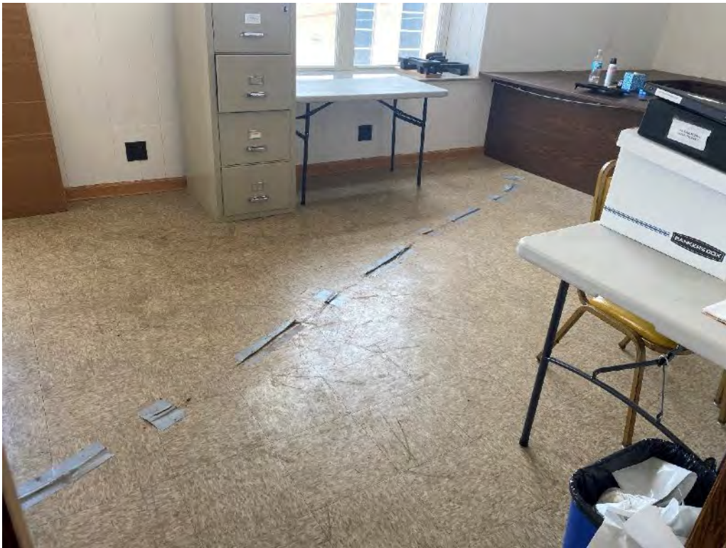
Asbestos Containing Black Mastic assoc. w/ 12"x12" Beige Mottled Floor Tile – Main Office
