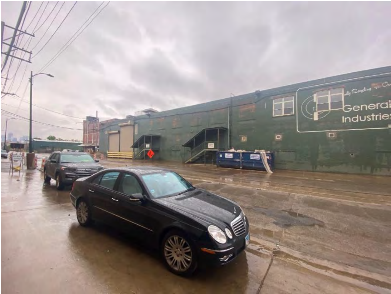
Photo 1 Existing Brick bearing wall along south face
