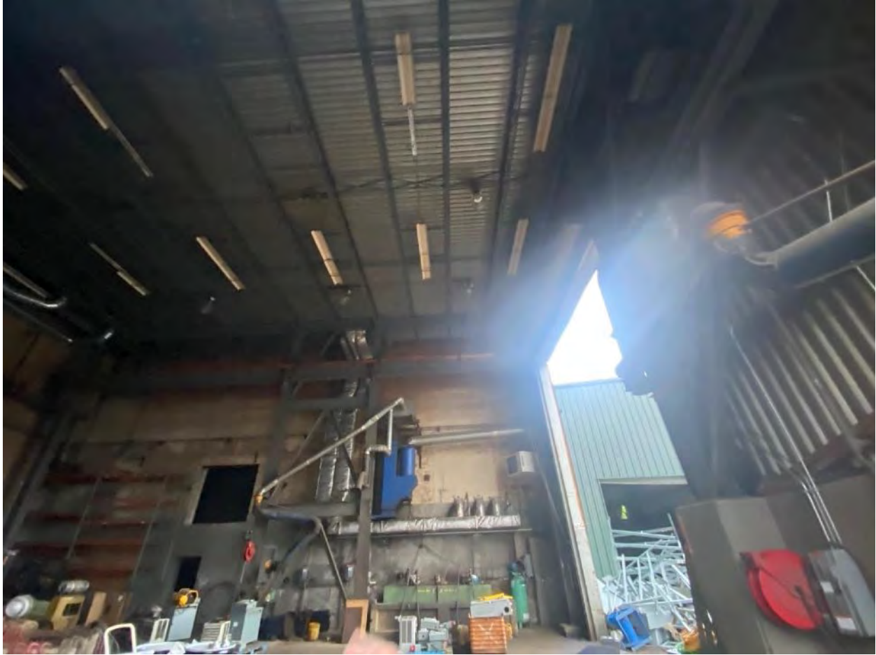
Photo 2 Typical high bay framing and interior bearing wall
