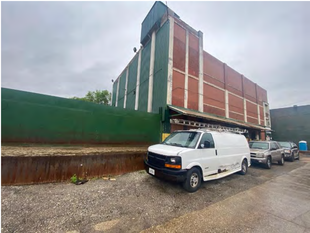
Photo 1 Existing Brick non-bearing brick wall along south and east elevations
