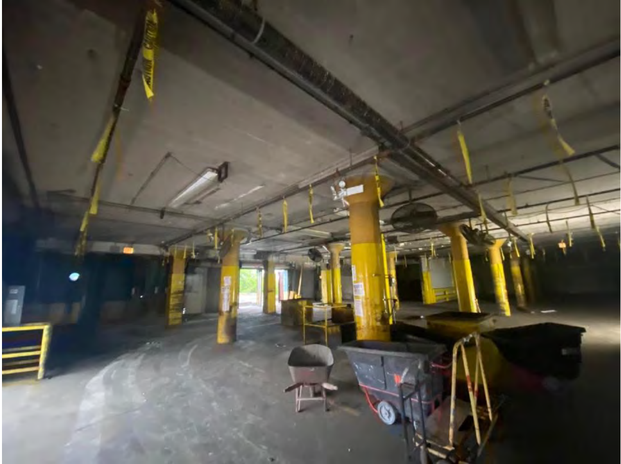
Photo 2 Typical bay framing
