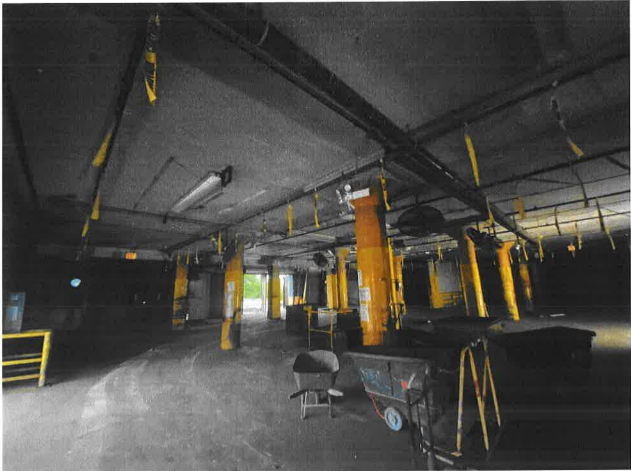
Photo 2 Typical bay framing
