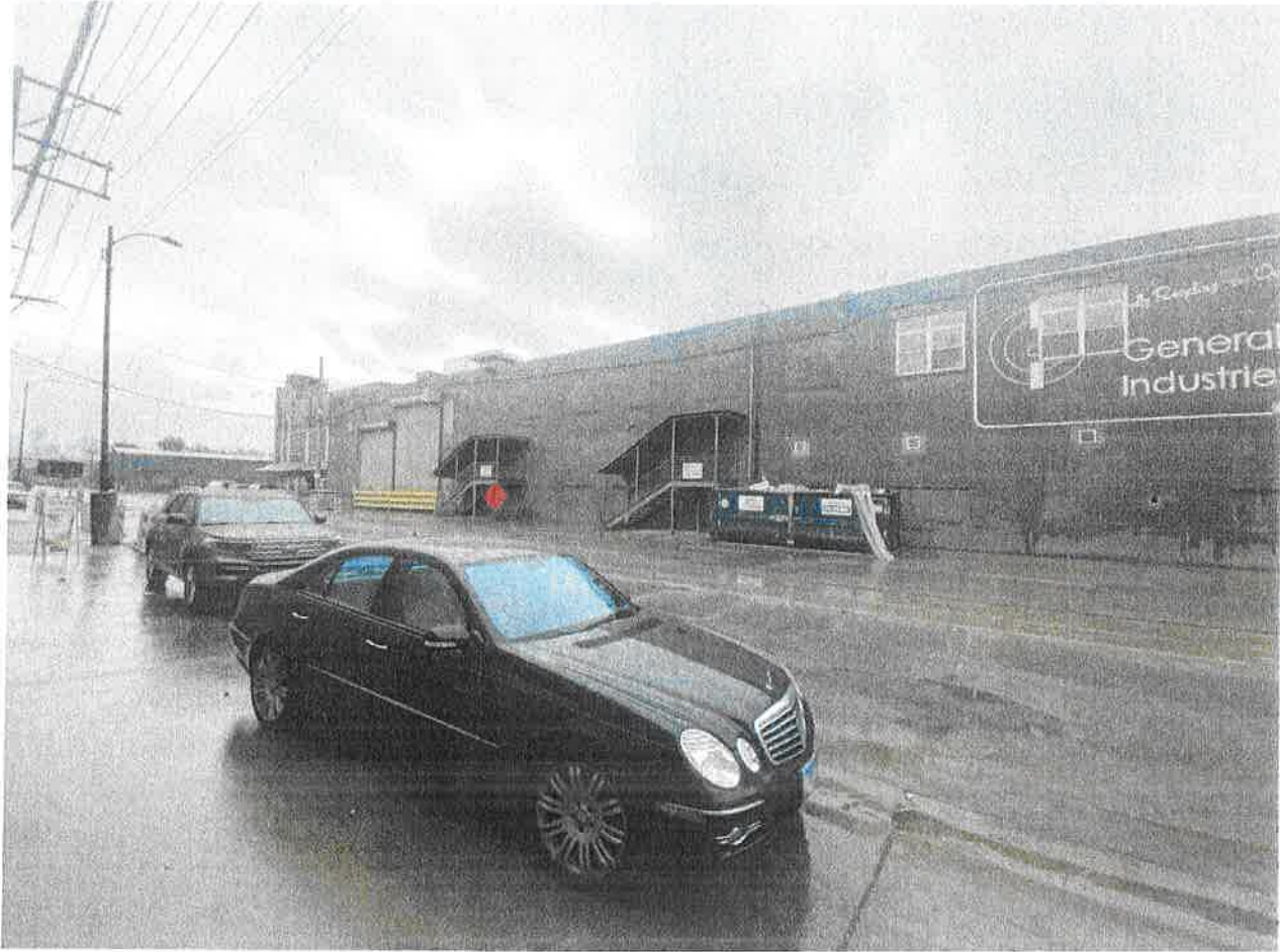
Photo 1 Existing Brick bearing wall along south face
