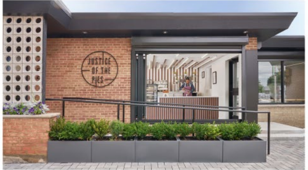
Justice of the Pies / Avalon - Completed, 2023
