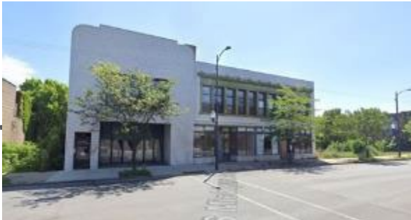
SITE #2 ROSELAND THEATRE
