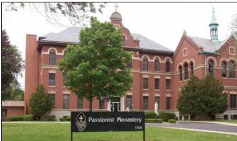
The landmark Passionist Brothers Monastery in the 41st Ward will be preserved and transformed into an affordable 84-unit senior complex.
