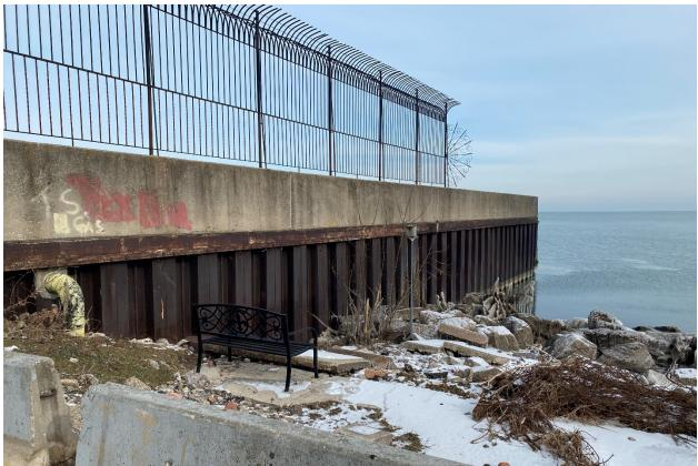
Photo 5 Steel sheet pile and concrete seawall, with rubblemound revetment in the foreground.
