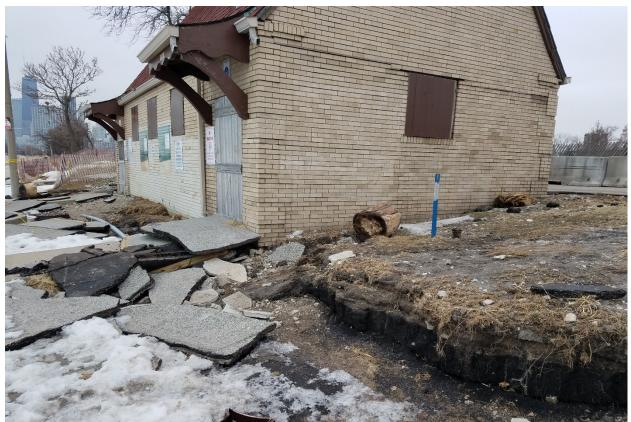
Photo 7 Erosion and storm damage to the lakefront trail at the historic North Avenue washroom facility.
