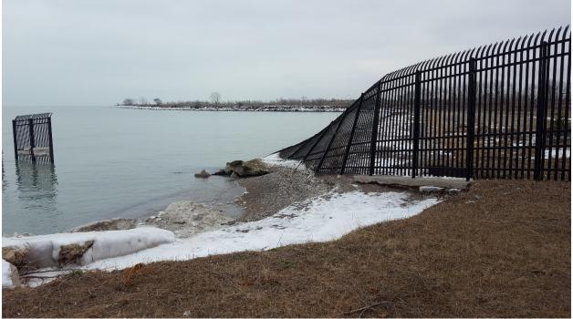
Photo 6 Erosion and fence damage as a result of the January 11, 2020 storm adjacent to the Eugene Sawyer Water Purification Plant
