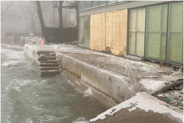
Photo 3 Storm damage to lakefront property, including broken windows, resulting in interior first floor flooding.
