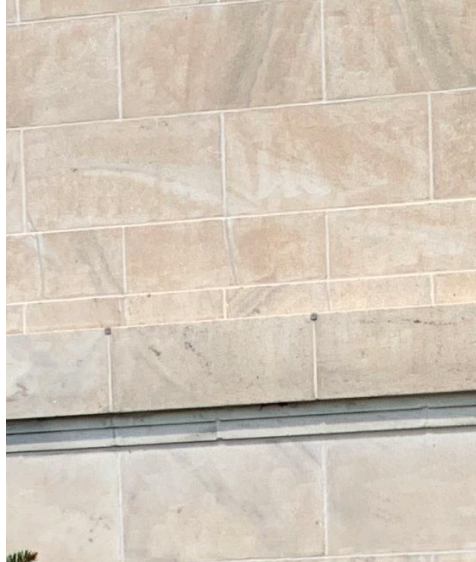
Existing Marble Façade: Georgian Marble
