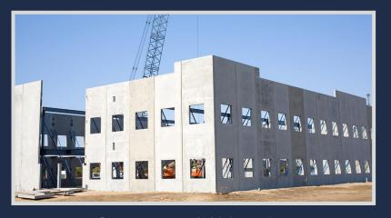
Precast concrete panel w/window openings
