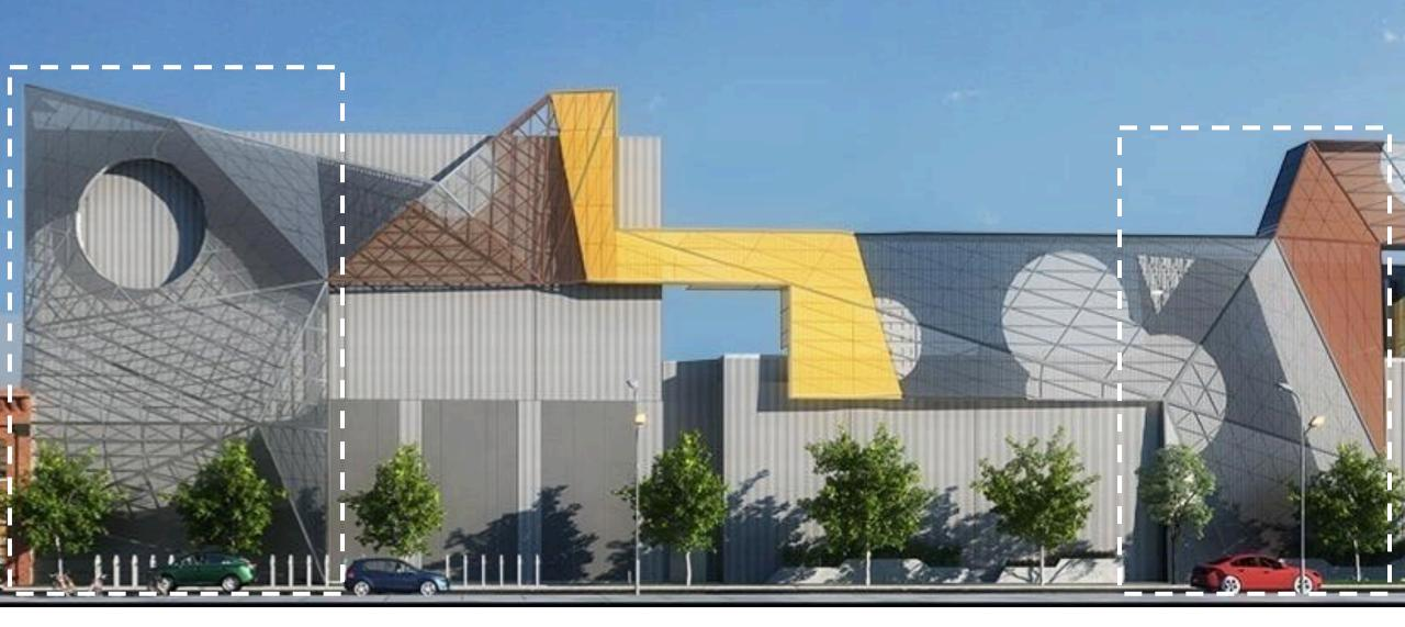
4. Pre-finished metal mesh screen extends to ground plan, in order to break up mass of Stadium and VR Arena spaces. Due to the programmatic requirements of backstage and VR Arenas, the Stadium and VR volumes cannot have windows. The screen will create light, shadow and texture at the pedestrian level.
