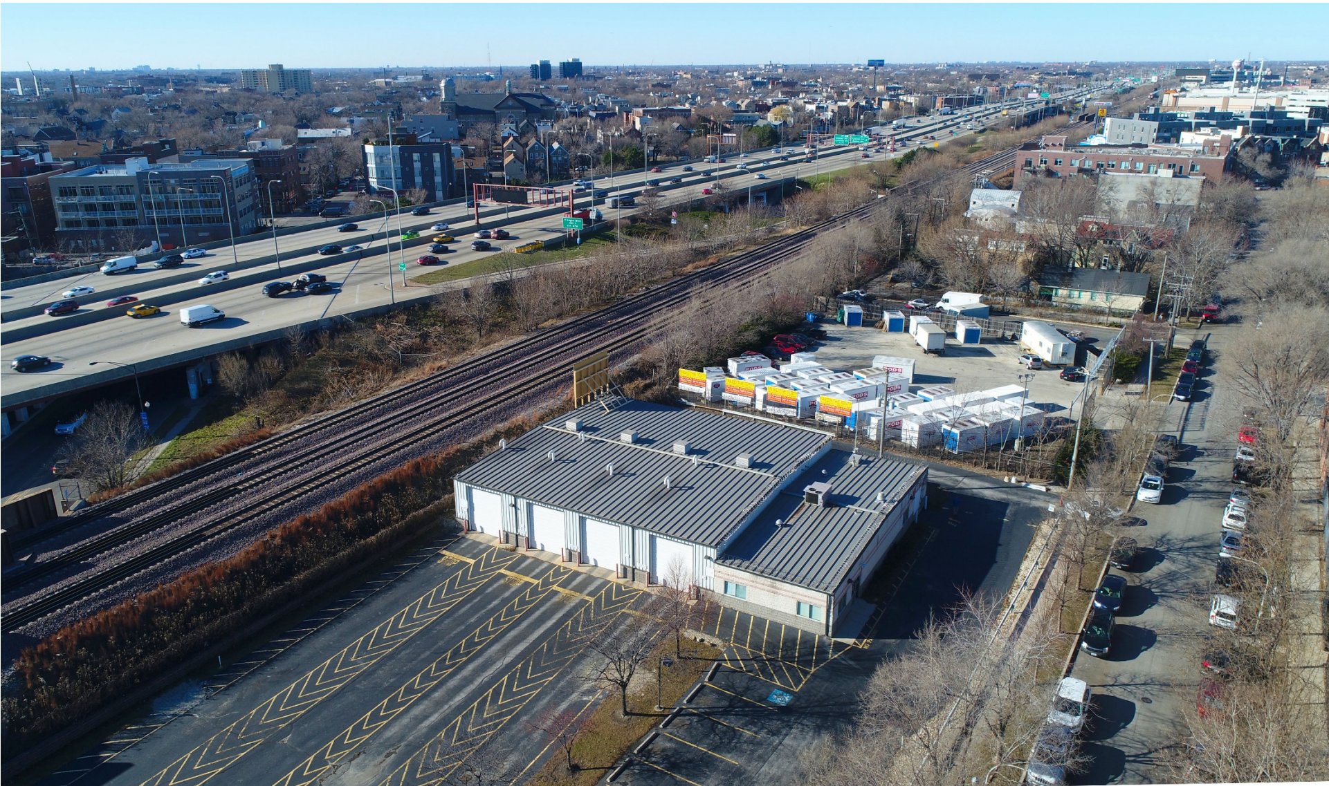
Existing Building Looking Northwest
