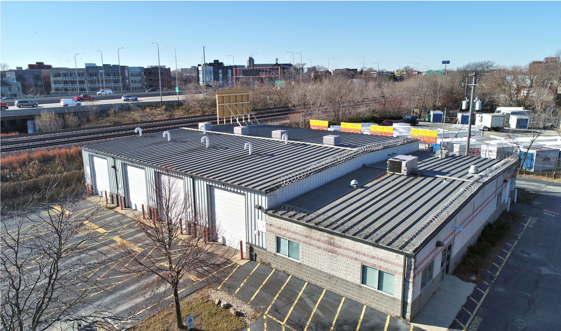
Existing Building Looking Northwest
