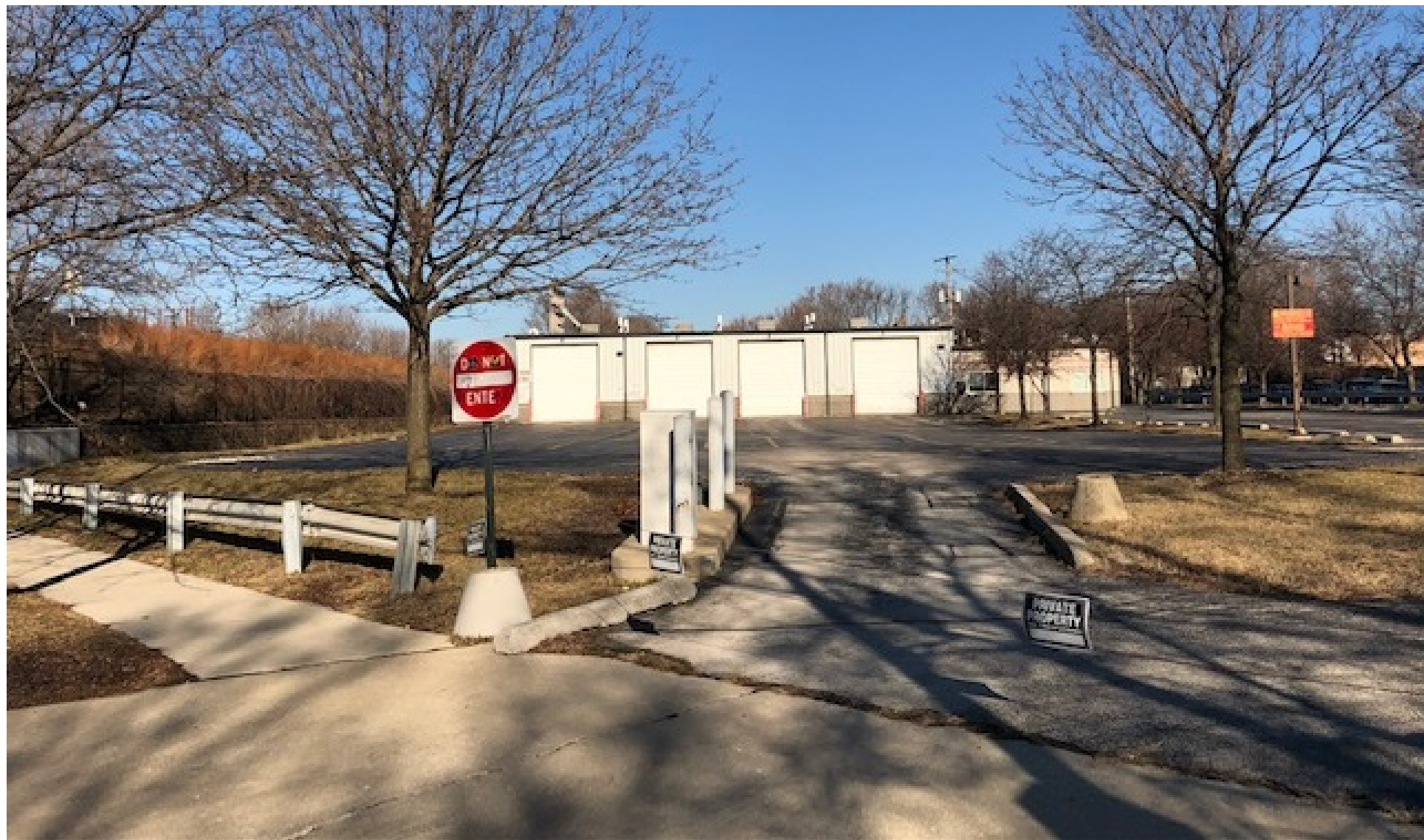
Existing Building South Elevation
