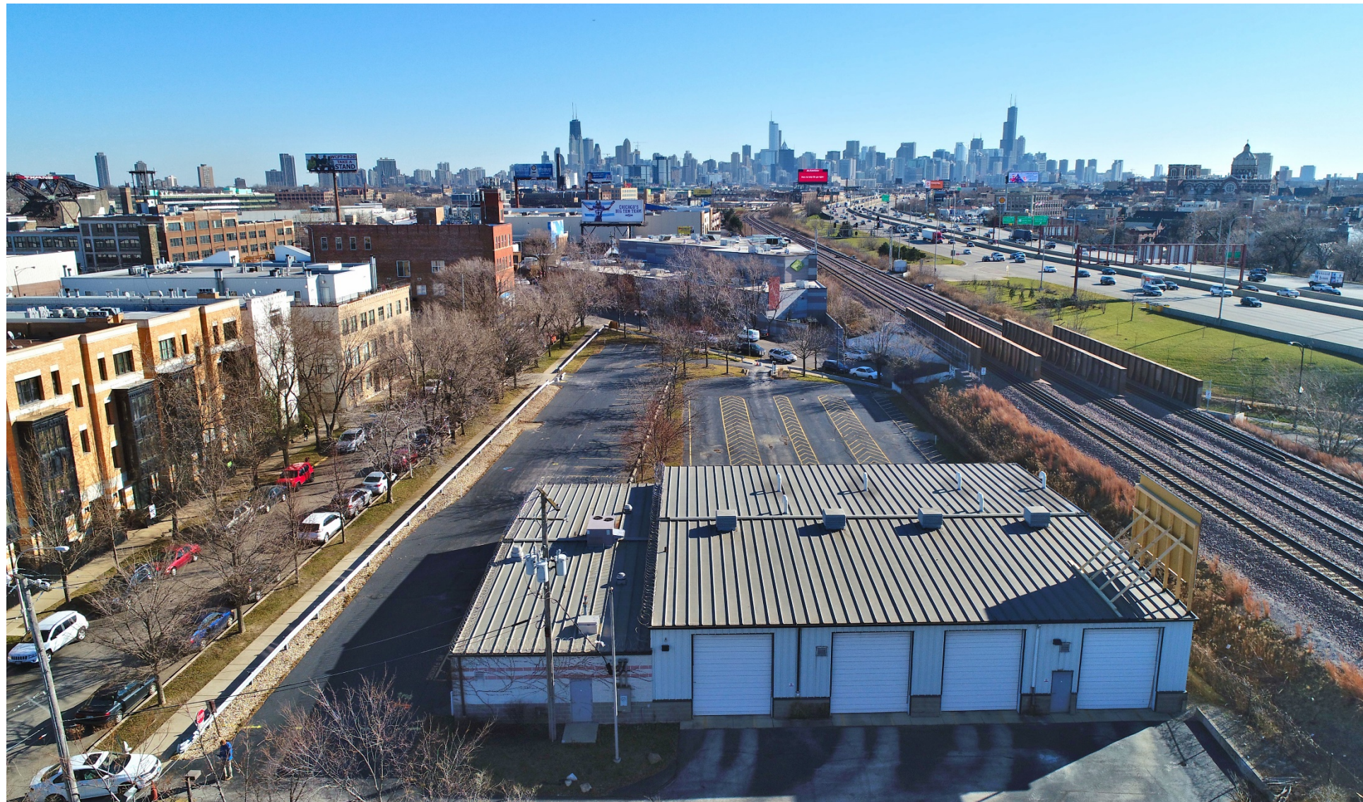
Existing Site Looking South
