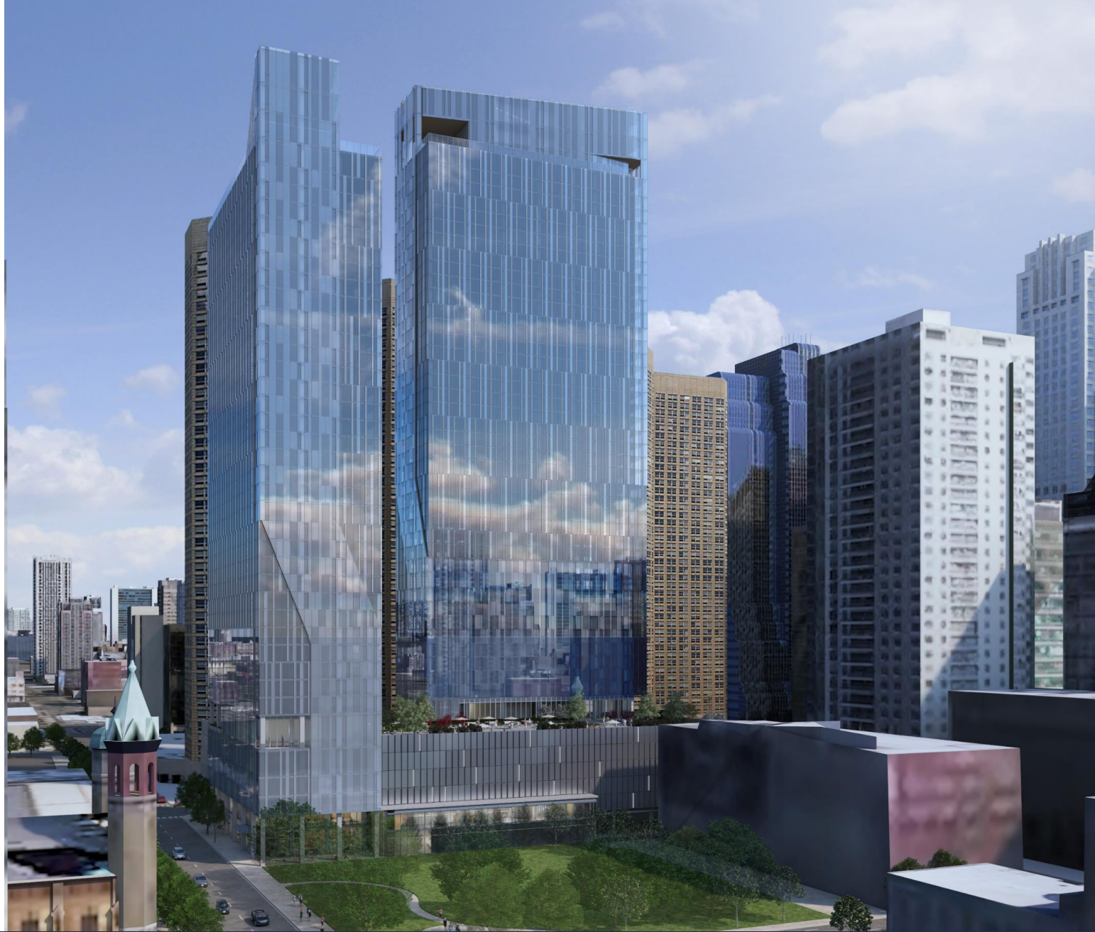
AERIAL VIEW FROM SOUTHWEST
