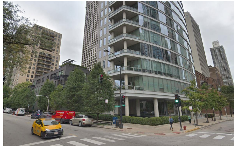
VIEW FROM DEARBORN ST LOOKING NORTH EAST
