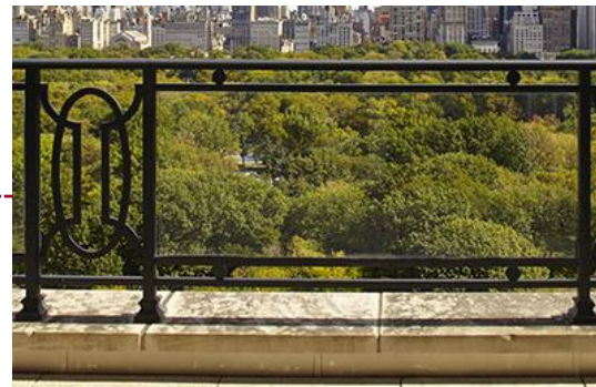
Glass & ornamental metal balcony
