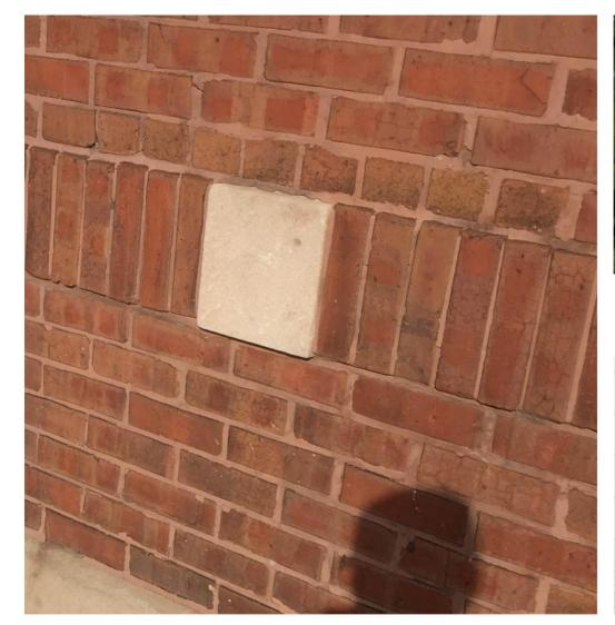
NEW MASONRY AND LIMESTONE SILLS TO MATCH EXISTING
