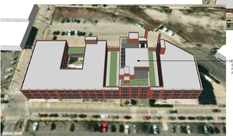
NEW ROOFTOP ADDITION EXISTING ROOF ELEVATION: APPROX. +48'-0" PROPOSED ADDITION PARAPET ELEVATION: 61'-3" PROPOSED ELEVATOR OVERRUN ELEVATION: 66'-3"
