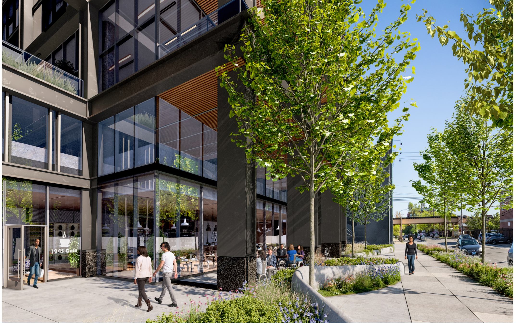
VIEW FROM NORTHWEST – LOOKING SOUTH DOWN N ELIZABETH ST
