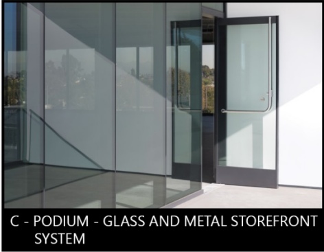
C - PODIUM - GLASS AND METAL STOREFRONT SYSTEM
