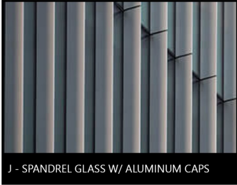
J - SPANDREL GLASS W/ ALUMINUM CAPS
