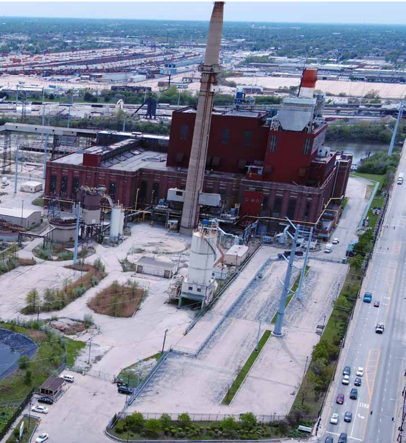
Crawford Power Generation Plant, Pulaski Road y 35th Street
