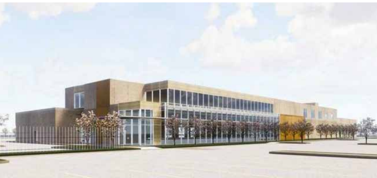
Peoples Gas Facility
