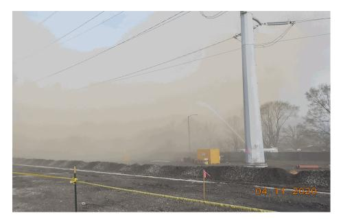
COMMENTS: Photo F- 3501 S. Pulaski Rd., Photo of dust cloud can be seen moving north onto residential area. Water truck can be seen hosing water.
