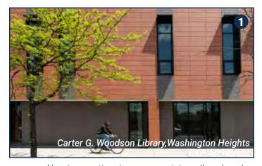
New terra cotta rainscreen curtain wall replaced a hazardous uninsulated brick facade that was falling apart
