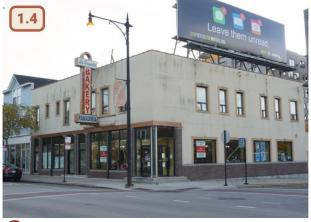
Figure 33. Unacceptable cladding over existing masonry
