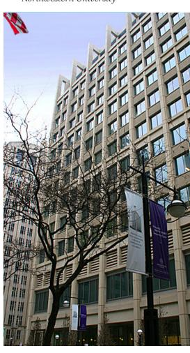
Built in the mid-2000s with a double skin facade and modern fixtures, envelope and lighting retrofits to the Lurie Medical Research Center provided only a marginal gain.
