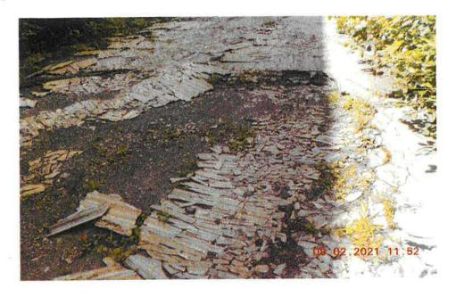
Photo E- 11600 S. Burley, Transite strewn across the roadway and ground following panel failure on north COMMENTS: side of the 32" building
