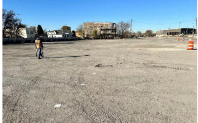
Photo 8: Utility clearing around B-15 prior to delineation sampling and remediation.
