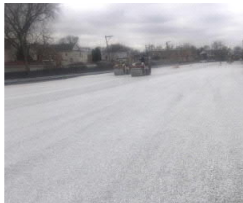
Photo 12: Installation completed of clean stone barrier throughout the site.
