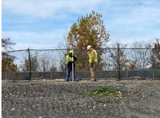
Photo 7: Typical temporary groundwater well installation.
