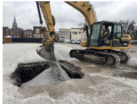
Photo 10: Backfill after removal of soil surrounding SB-15.
