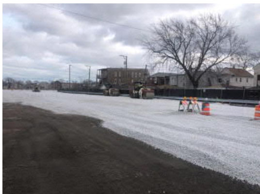
Photo 11: Spreading compacting of clean stone barrier.
