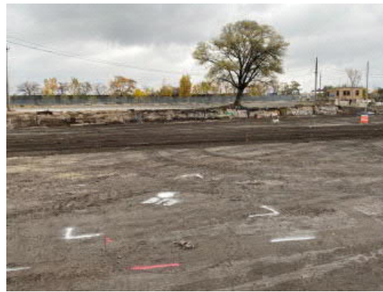
Photo 2: Typical boring marked and cleared for underground utilities.
