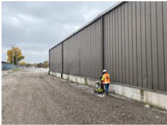
Photo 1: Private utility locating performed on the northern portion of the site.
