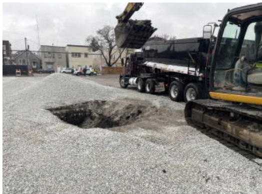
Photo 9: Loading soil surrounding SB-15 into a truck for offsite disposal.
