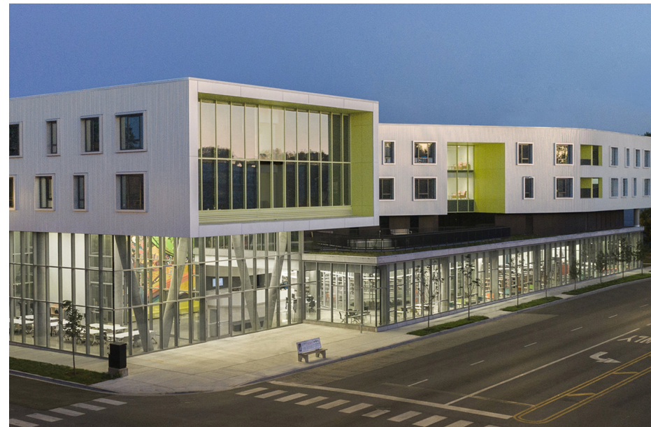
Northtown Branch Public Library at Western and Pratt Architect: Perkins and Will
