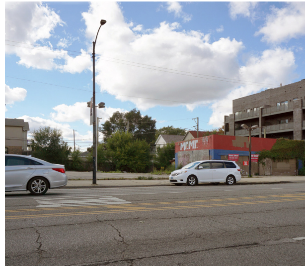
1F Vacant building/lot 3806-3816 N Western
