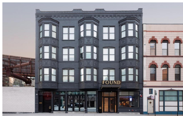
Found Hotel Chicago Source: Timeout Chicago, designed by NORR
