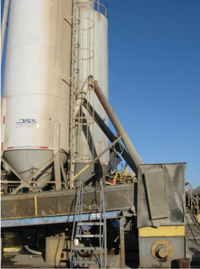
Cement storage silos at SA Bakersfield.
