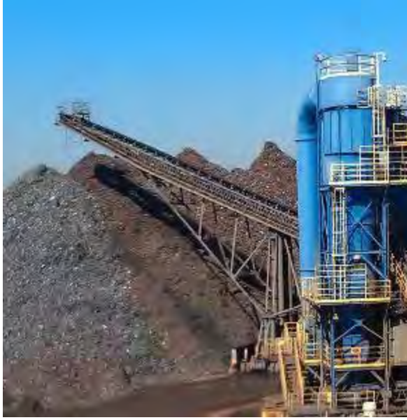
Pile of sorted ferrous metal following shredding of scrap metal at SA Terminal Island.
