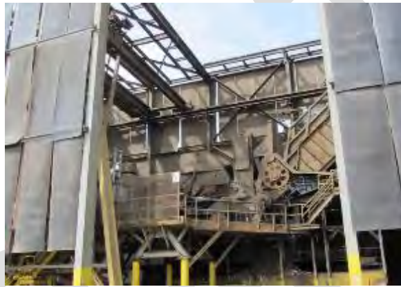
Shredder and loading equipment at Schnitzer Steel, Inc., Oakland, CA.
