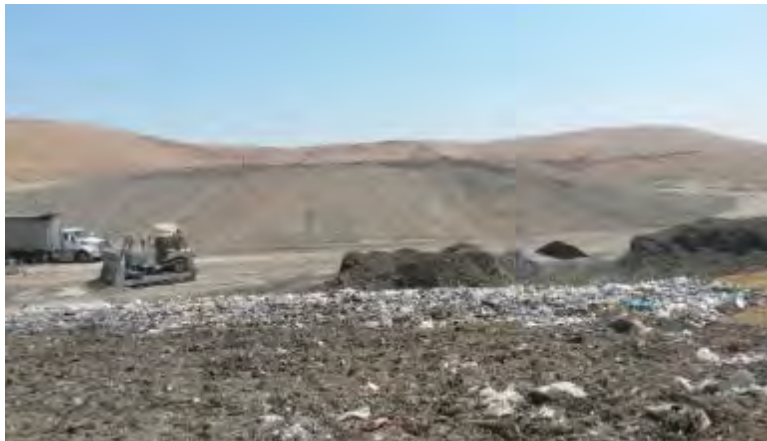
Vasco Road Landfill, Livermore, CA with municipal solid waste in the foreground (lighter material) and stockpiled CTMSR in the distance (darker colored material).
