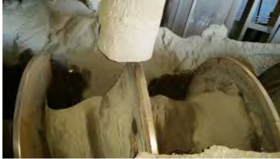
Tube for feeding cement into the pug mill for chemical treatment of metal shredder residue, Sims Metal Management, Redwood City, CA.
