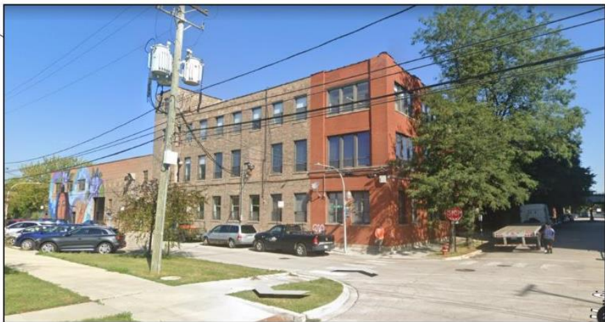
EXISTING CONDITIONS ALONG KINZIE AND MAY LOOKING NORTHWEST
