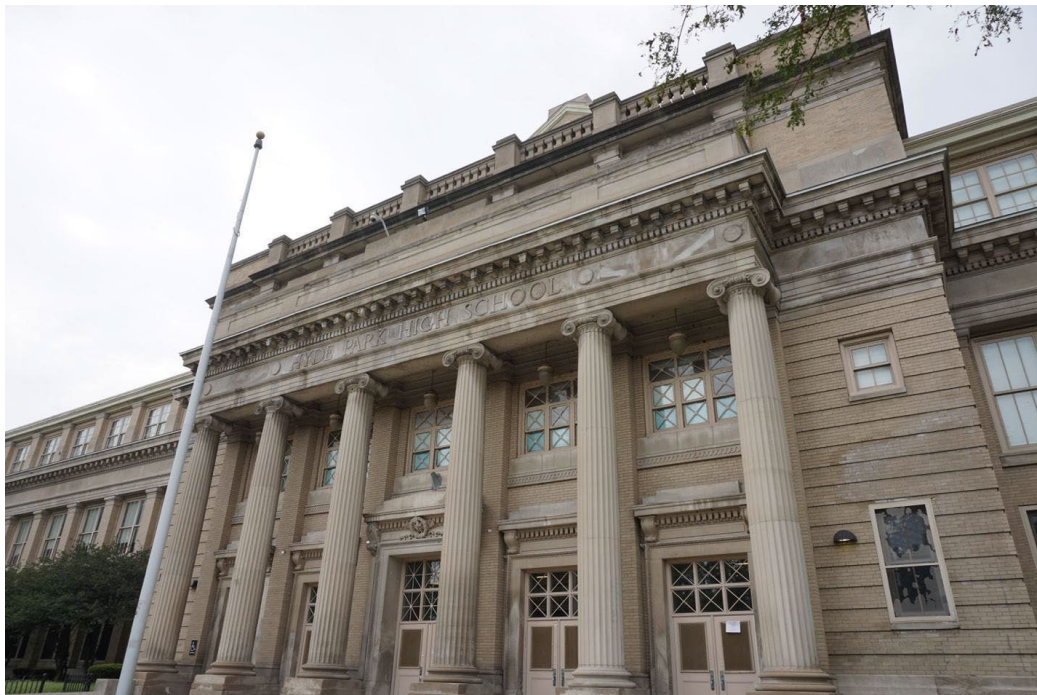
Photo 4: Hyde Park High School/Academy looking Southwest from S. Stony Island Avenue
