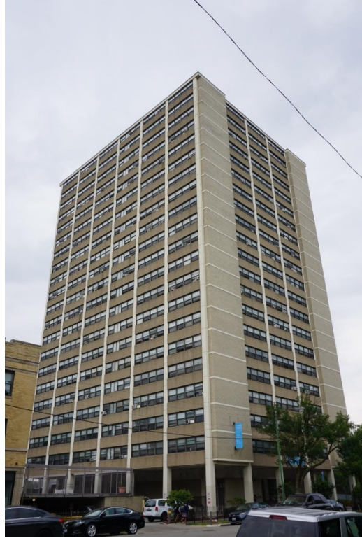
Photo 1: Island Terrace Apartments, 6430 S. Stony Island Avenue, view looking southwest from Stony Island Avenue of the north and east facades
