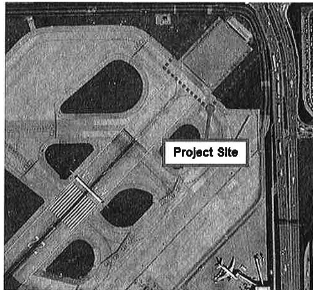
Figure 1-2. EMAS Location (22L Numbered End)
