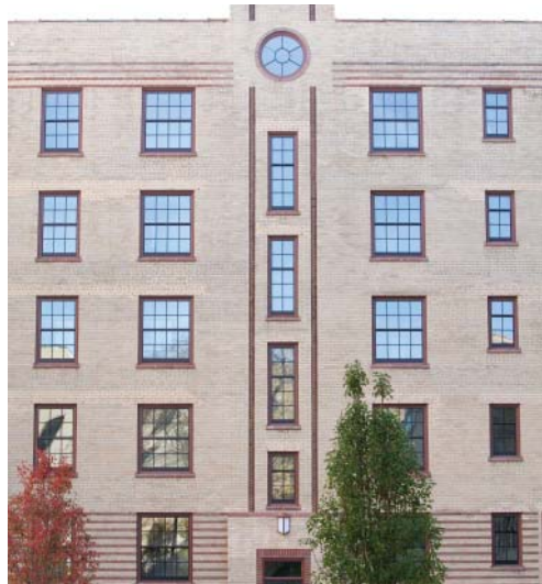
Facade (Credit: Chris Moe Photography)
