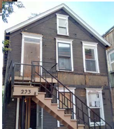
after siding removed
