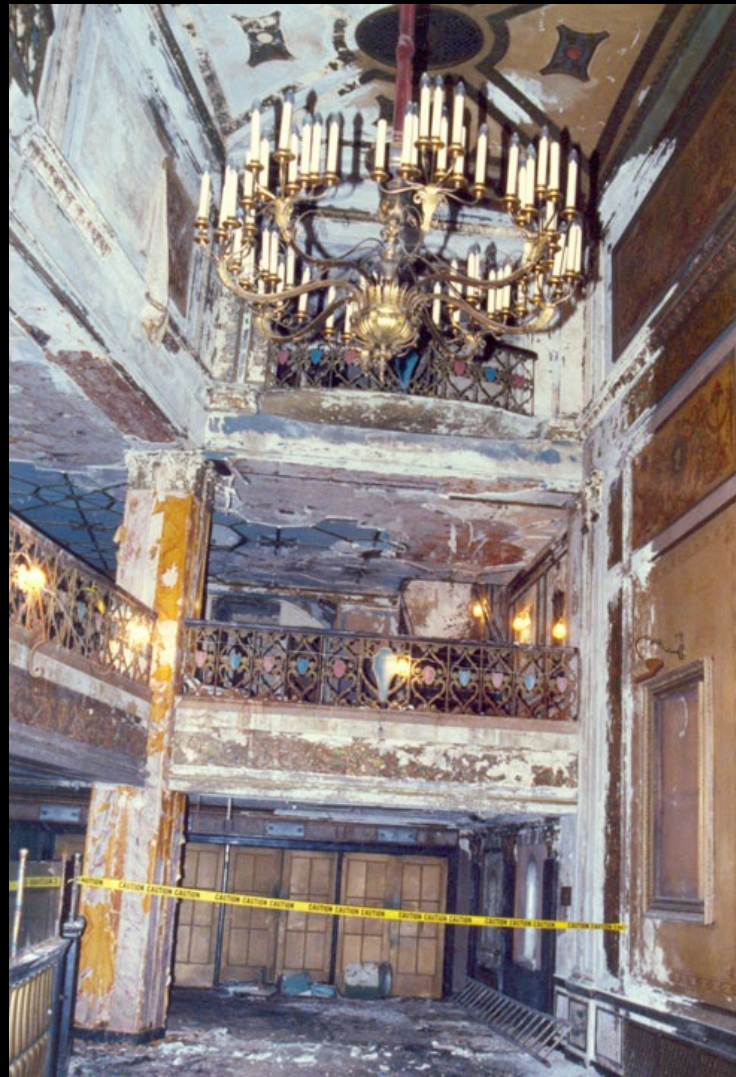
Detroit Opera House Before and After
