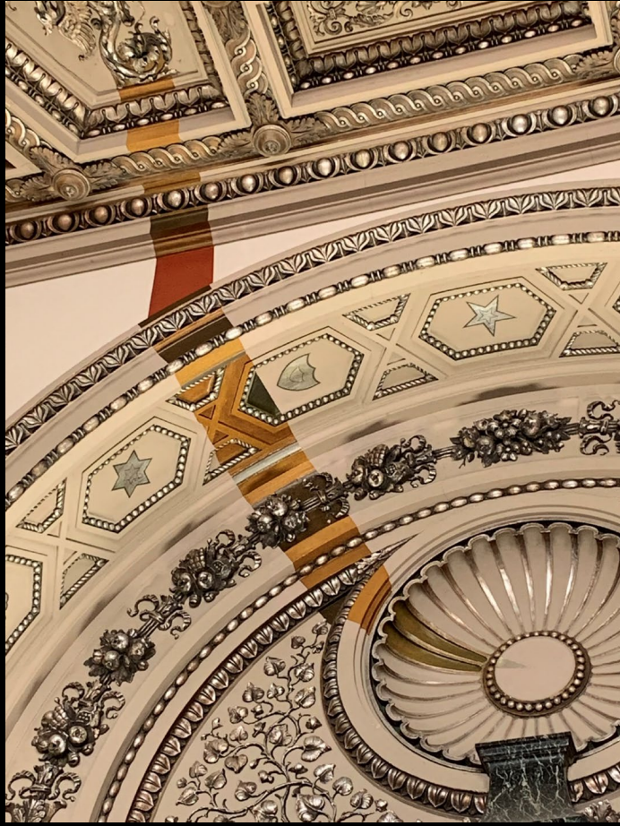
Test Paint Removal Strip
