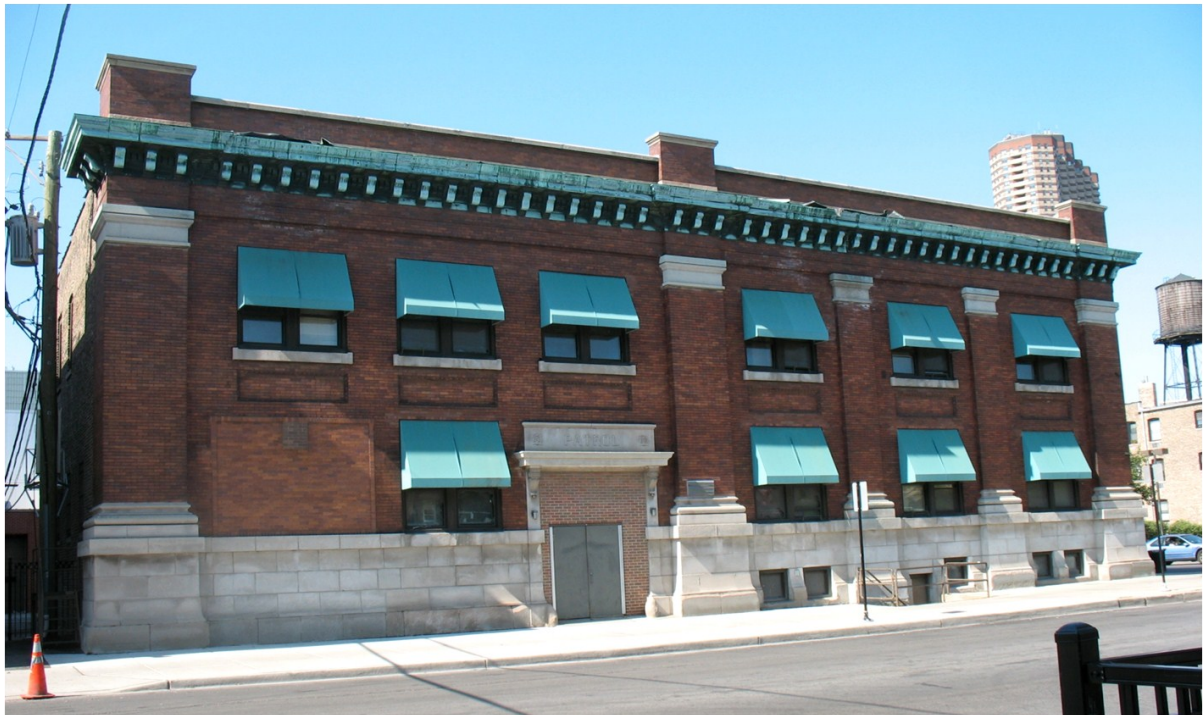
The 42nd Precinct / Town Hall Police Station is two-stories in height and built of brown brick and limestone trim. Top: A view of the building's Halsted Street façade. Bottom: The Addison Street façade.
