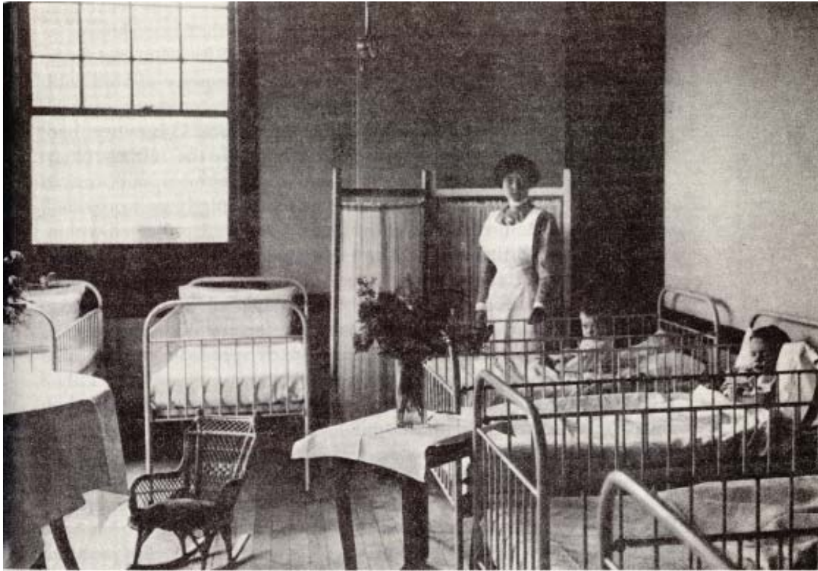
The Asylum Building also contained a kindergarten (top) and an infirmiry (bottom).
