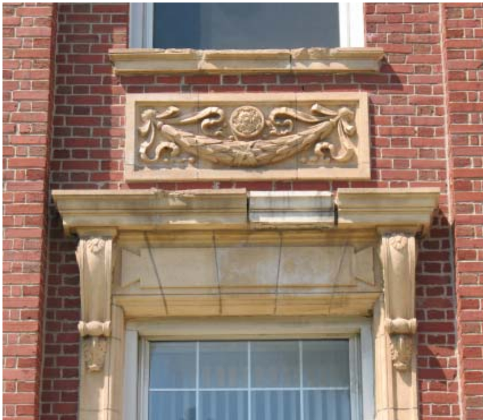
Photos of the Building's Classical-style ornament.
