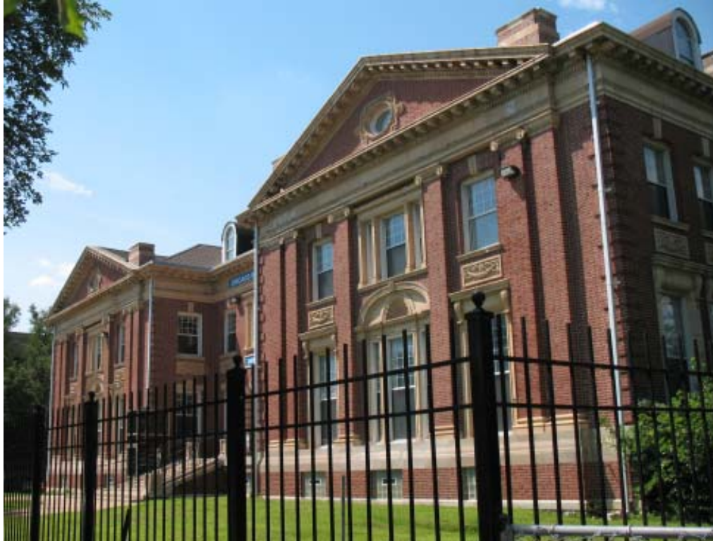
Top: The Chicago Orphan Asylum Building is 2 1/2-stories in height and designed in the Colonial Revival architectural style. Red-brick walls are ornamented with brick Ionic pilasters and terra-cotta cornices, window surrounds, and spandrel panels.
