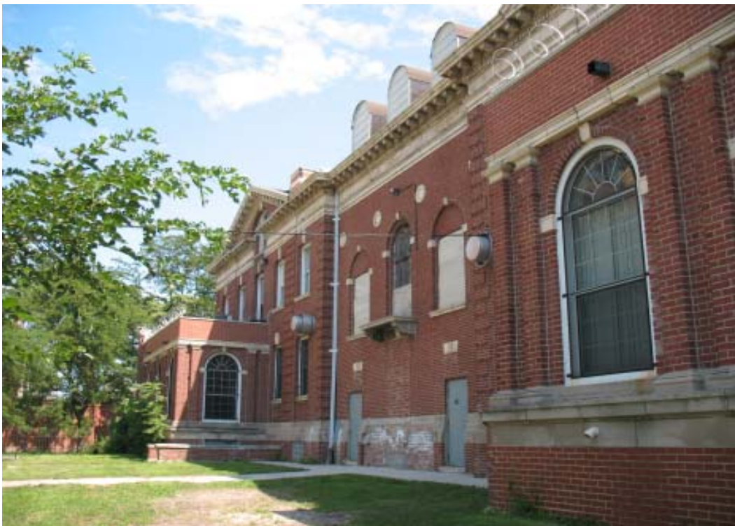
Top: The side elevations are similarly decorated with brick pilasters and Classical-style terra-cotta ornament.
