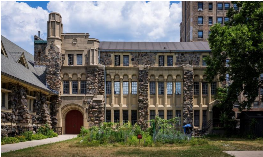
The front façade of the community house includes an entrance bay topped with Gothic Revival towers and a Romanesque arcaded corbel band above the second floor windows.
