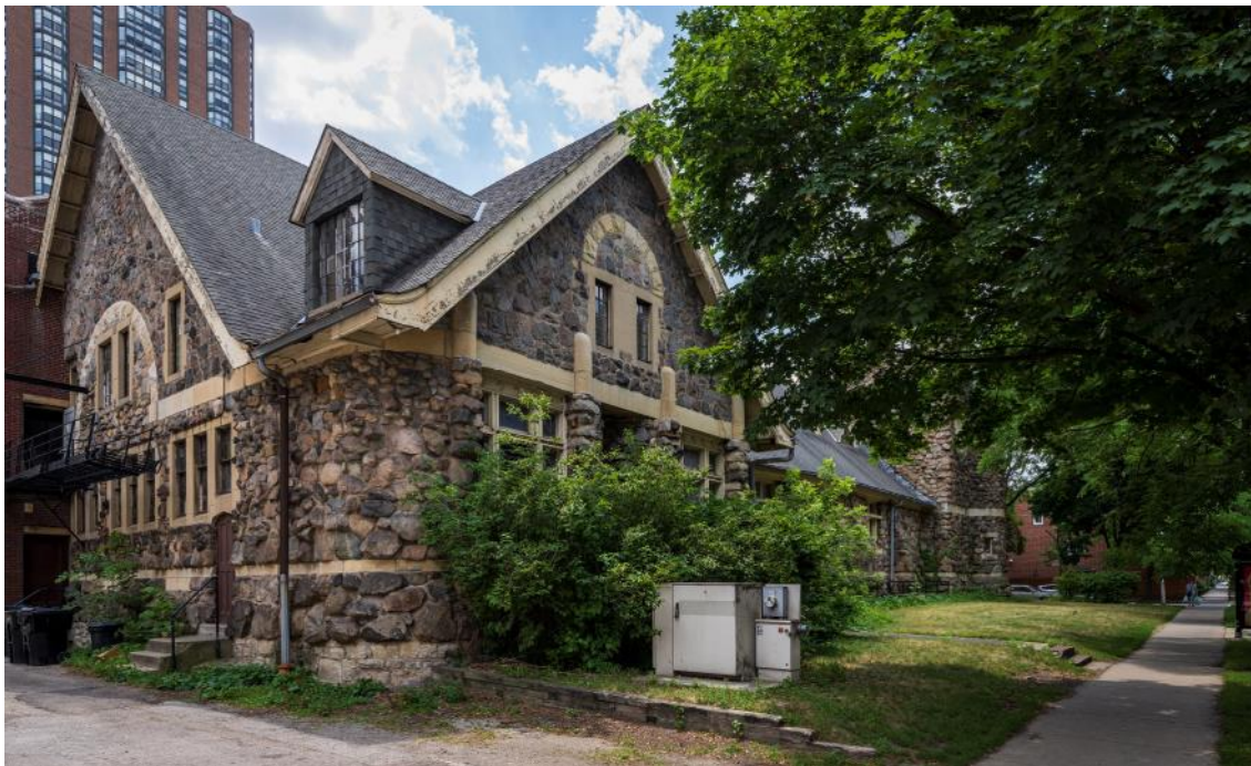
The right gable in this photo is the cross gable forming the T-shape at the east end of the church. The left gable is the rear of the church facing the alley and faced in stone
