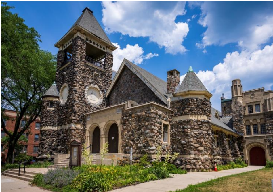
Epworth 2022, showing the addition of the narthex and a partial view of the community house addition which are historically significant changes.
