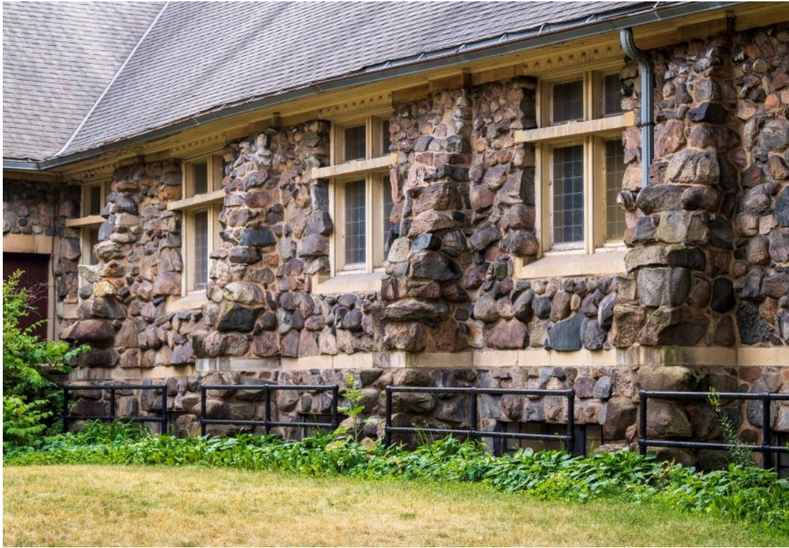
The side elevations of the church building feature buttresses dividing the wall into equal bays each with a pair of casement and transom windows,
