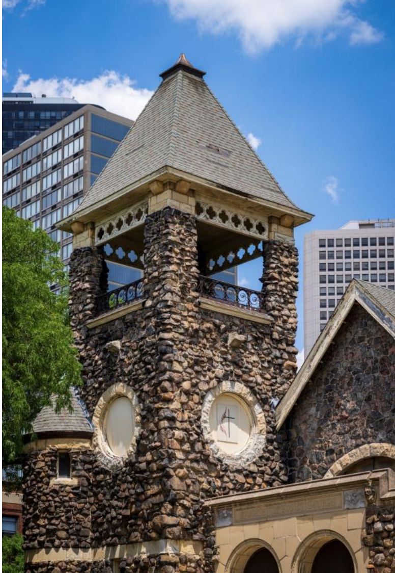
Detail of the 65-foot-tall square tower with the round turret bracing its corner. The oculus windows are boarded up, but the circa 1960 photo below shows that these openings contained quatrefoil tracery.
