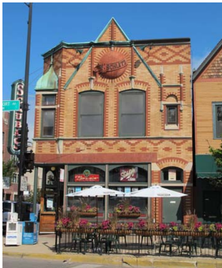
(Former) Schlitz Brewery-Tied House (now Schuba's Tavern) 3159 N. Southport Ave. Date: 1903 Architect: Frommann & Jepsen
