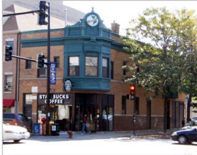
(Former) Schlitz Brewery-Tied House 2159 W. Belmont Ave. Date: 1903-04 Architect: Charles Thisslew
