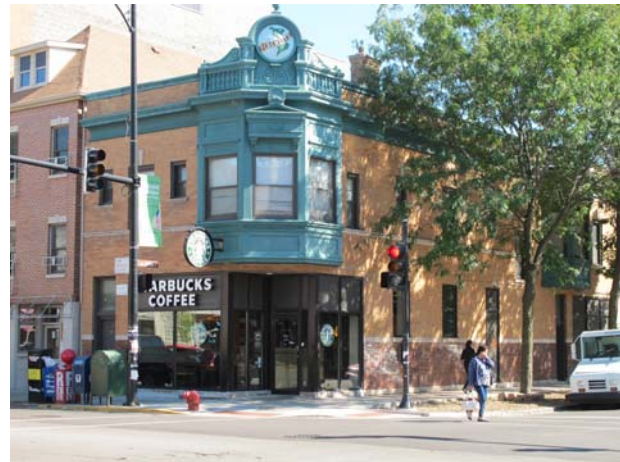
(Former) Schlitz Brewery-Tied House 2159 W. Belmont Ave. Date: 1903-1904 Architect: Charles Thisslew
