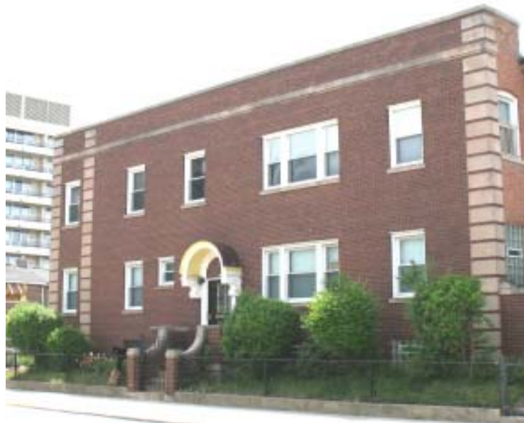
Right: The Anderson house at 3800 S. Calumet Ave. displays the influence of the Colonial Revival style with its round-arched pent roof over the front door and its stylized limestone quoins that visually define the building's corners.
