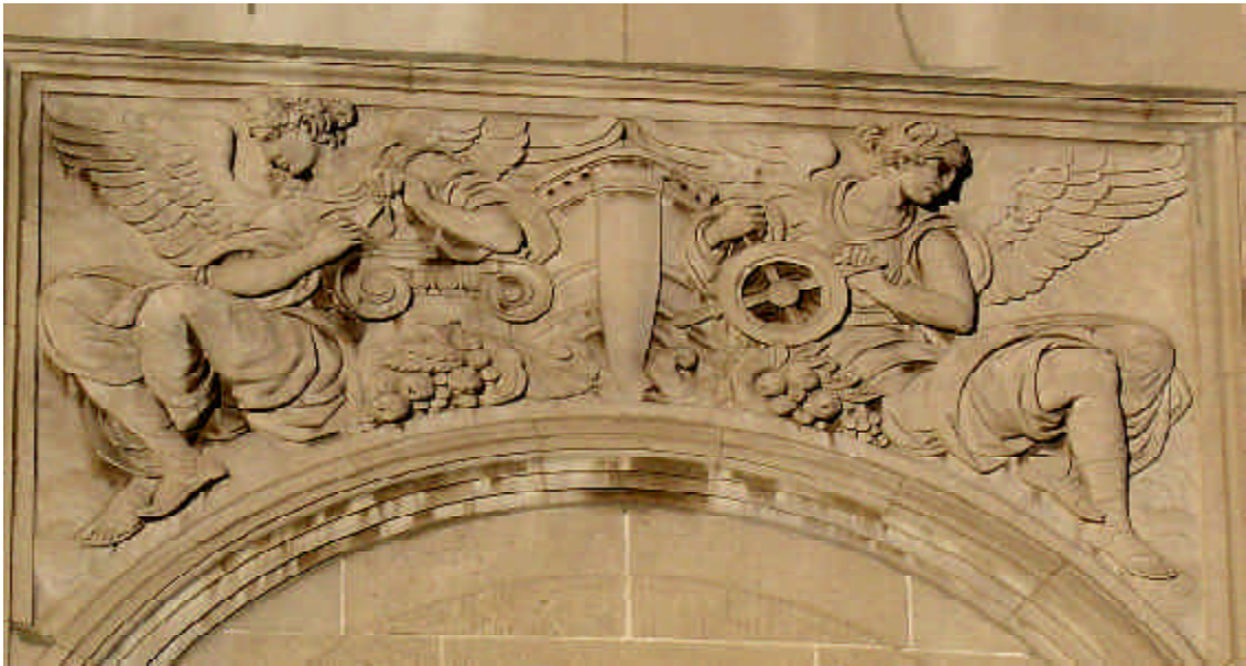
The building's exterior is ornamented with well-crafted Classical-style decoration, including (top) angels flanking a medallion over the main banking entrance and upper-floor pilasters and pediments; and (bottom) allegorical figures above the now-blocked ground-floor windows.
