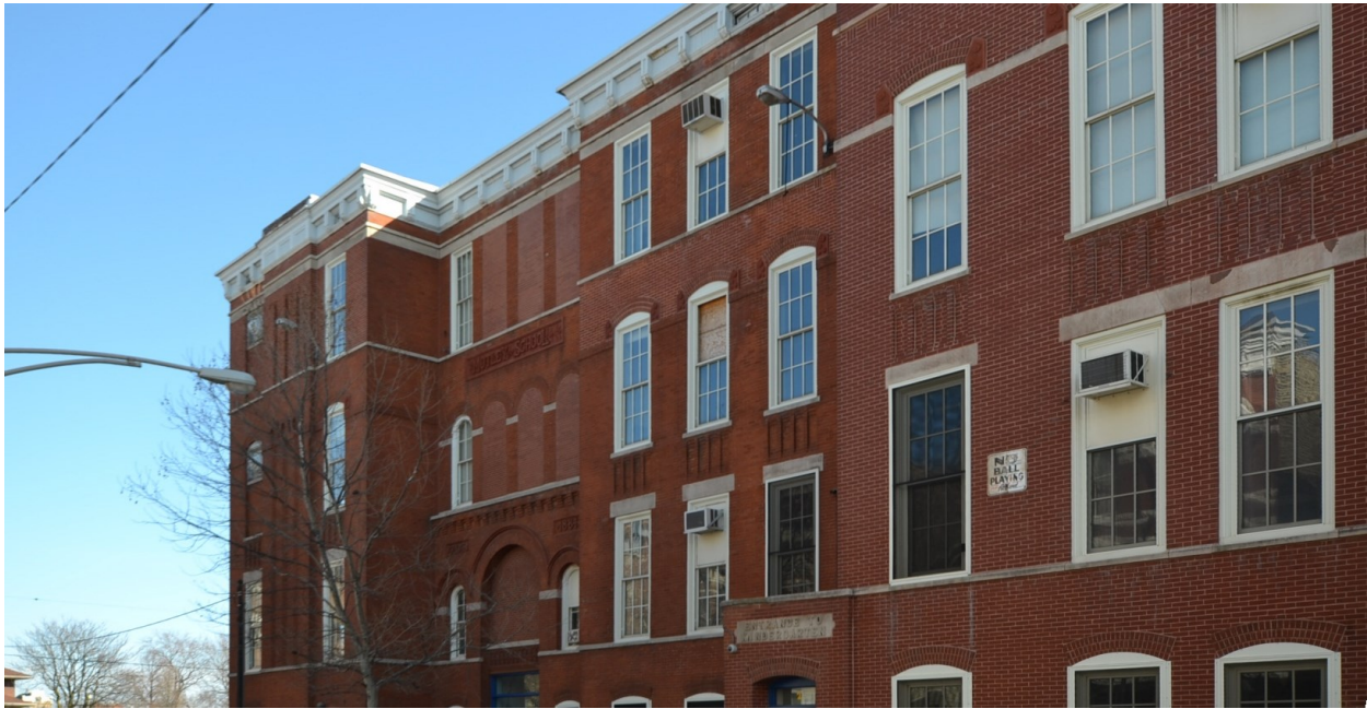
The Motley School was built in 1884 (left) with a seamless addition completed in 1898 (right).
