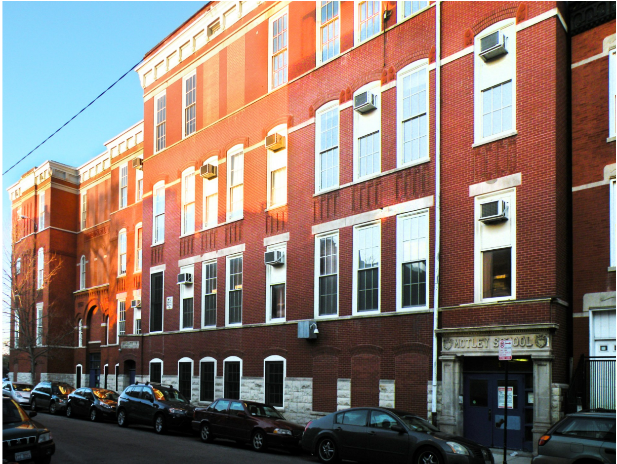
Image 8: Normand S. Patton's 1898 addition to the Motley School matches Flanders's original 1884 design in its materials, design, and details.
