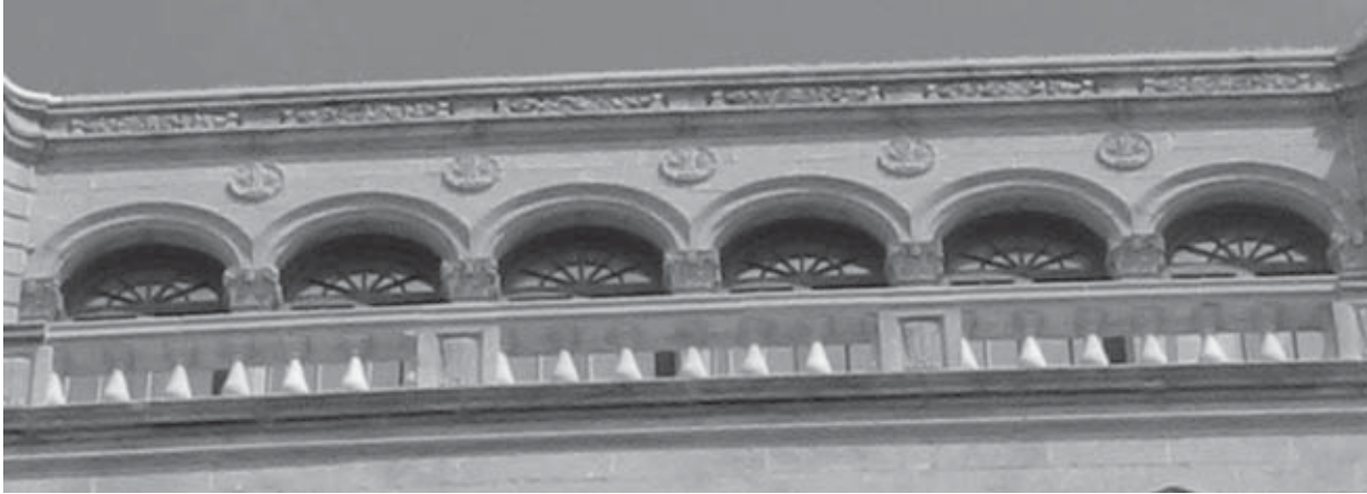
The North Chicago Hospital Building is crowned with a solarium that features arcaded french doors set back from the facade behind a continuous balustrade.
