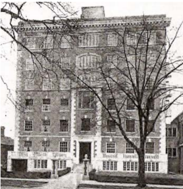
Typical of the need for hospital beds as the U.S. population increased was the Harbin Hospital (left) in Rome, Georgia. A new 40-bed hospital was erected in 1917, but only three years later the town found it necessary to add three stories, for an additional 35 beds. The local architects brought Sturm in as a consultant for the rooftop addition, seen in this photograph.
