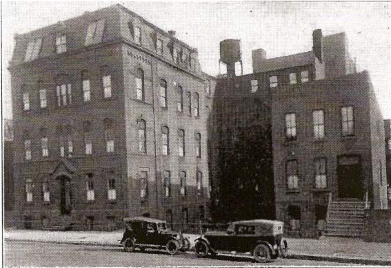
Passavant Memorial Hospital (above) was founded with the medical needs of poor immigrants in mind. (This building in the 100-block of W. Superior has been demolished.)
